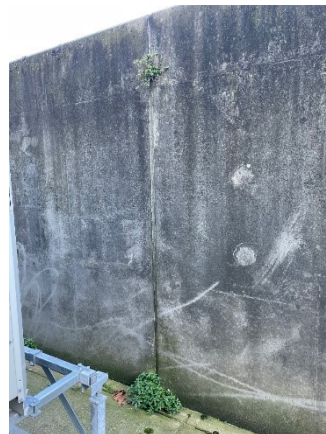
24 – River face rear movement joint
