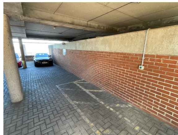
27 – Car park under-croft brick face
