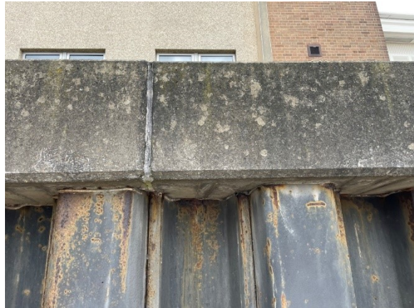
8 - Riverside capping beam movement joint
