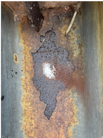
15 - UMT inspection example
