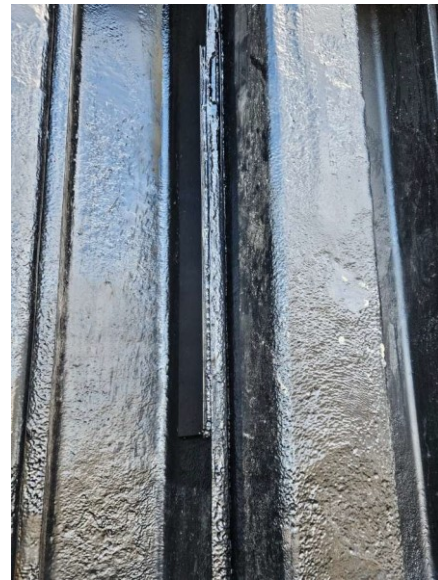
32 – Steel plate repair
