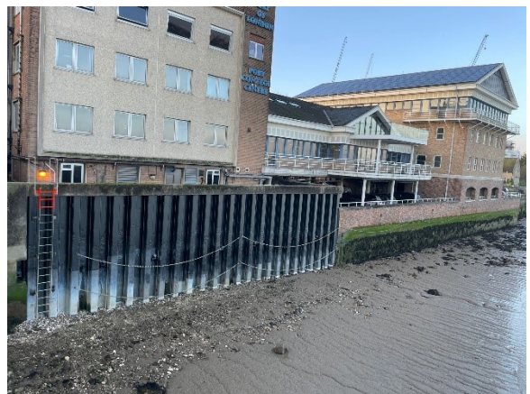
28 – LW following remedial works – note discolouration of piles due to saline water reacting with paint dye. The coating has not been compromised.
