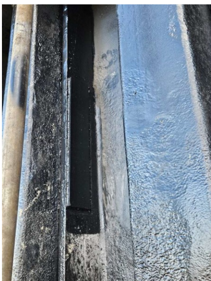
33 – Steel plate repair
