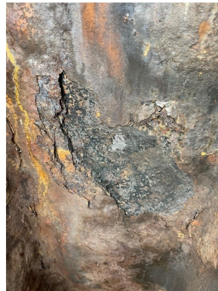
16 - UMT inspection example
