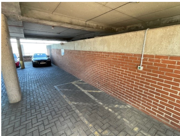
5 - Car park face front
