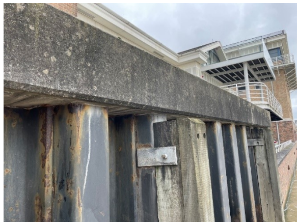
6 - Riverside capping beam
