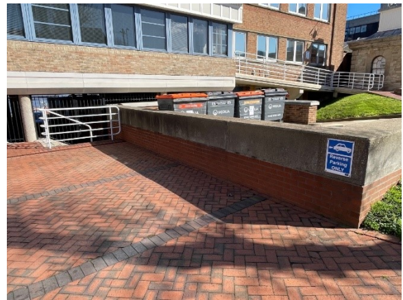
28 – Bin store car park brick face
