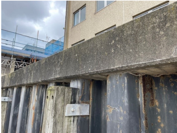
7 – Riverside capping beam
