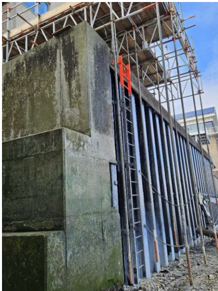
31 – LW following remedial works
