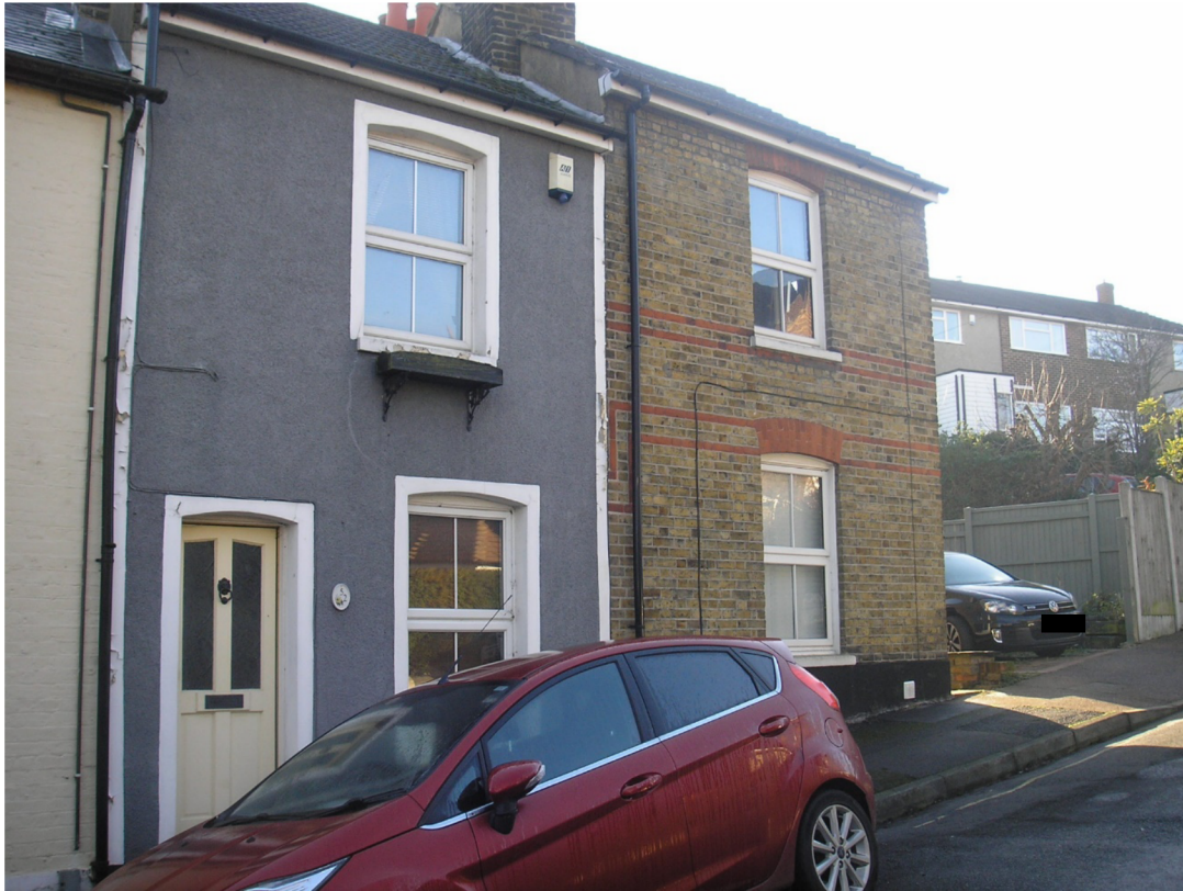
3 Nos 52 and 53 with Nos 59 and 60 in background
