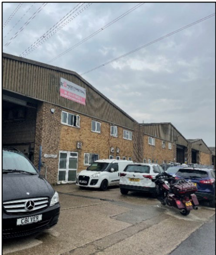
Buildings located in the north-western portion of the red line boundary
