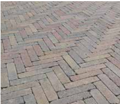
Clay block paving
