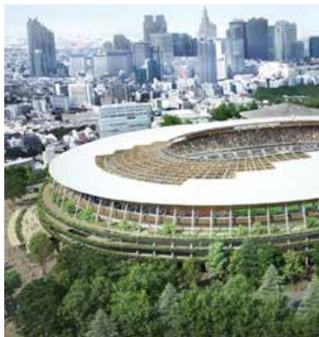
Japan National Stadium - Kengo Kuma
