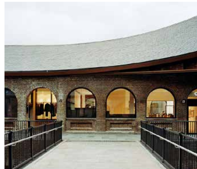
Coal Drops Yard - Heatherwick Studio
