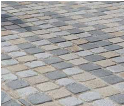
Tumbled vehicular sett paving, buff tones
