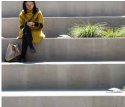
In situ grey concrete, polished
