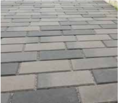
Permeable vehicular sett paving,
