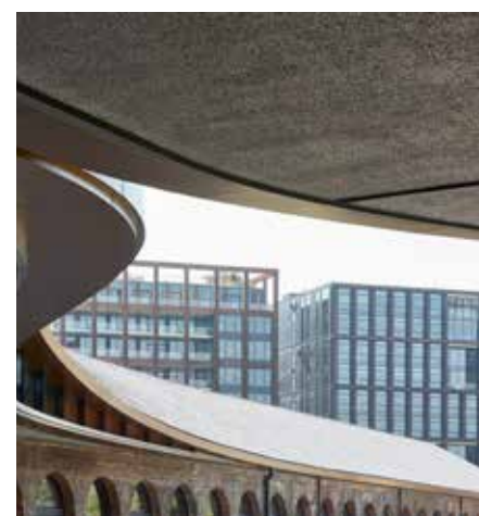
Coal Drops Yard - Heatherwick Studio
