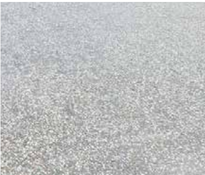
In situ exposed grey aggregate poured concrete
