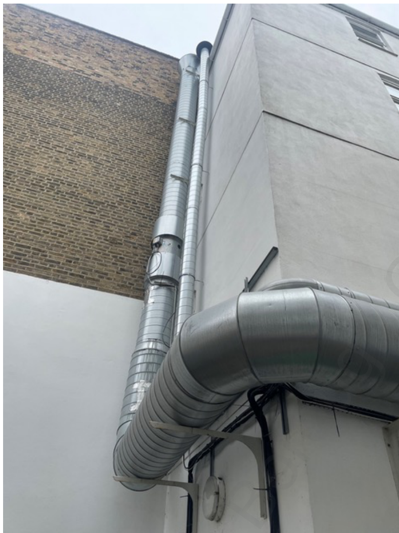
FIGURE 5: EXTERNAL EXTRACT FLUE 1M ABOVE ROOF
