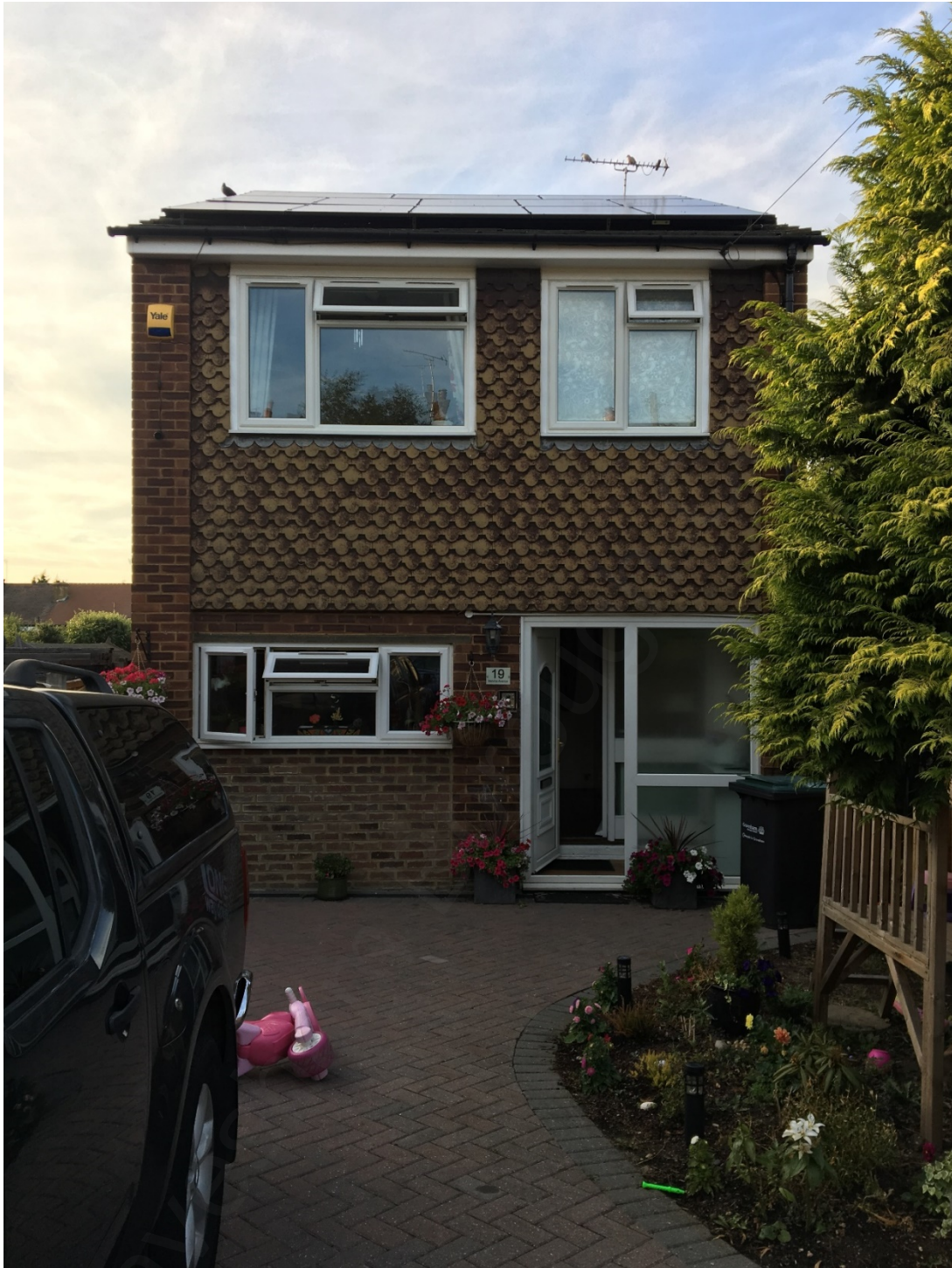
Existing front elevation with finished brickwork at ground floor level and tiled façade at first floor level.
