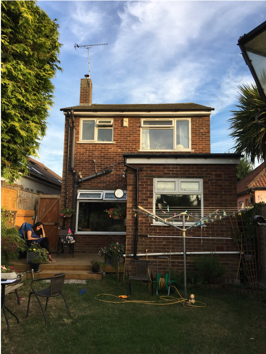
Existing rear elevation, all finished faced brickwork.
