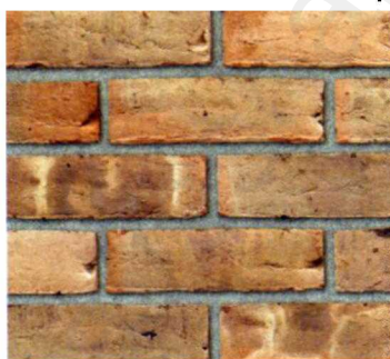
Buff/ Reds facing stock brickwork
