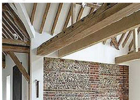
Lime render with brick quoins and flintwork
