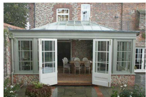
Timber frame orangery
