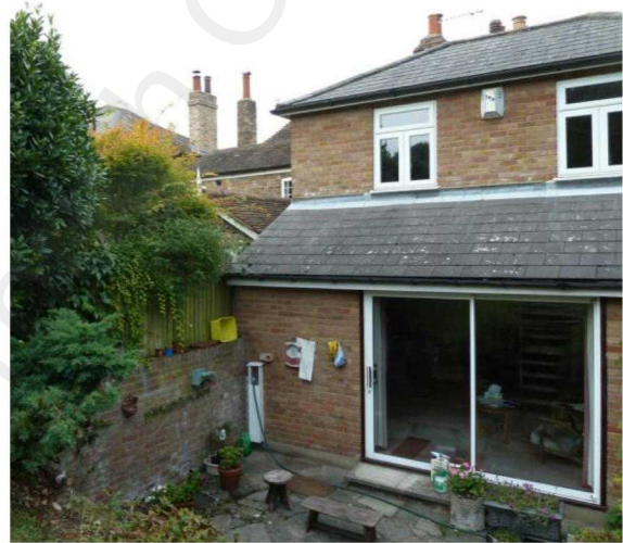
View 5 – Old Pump Cottage rear view in context with Ivy Cottage.
