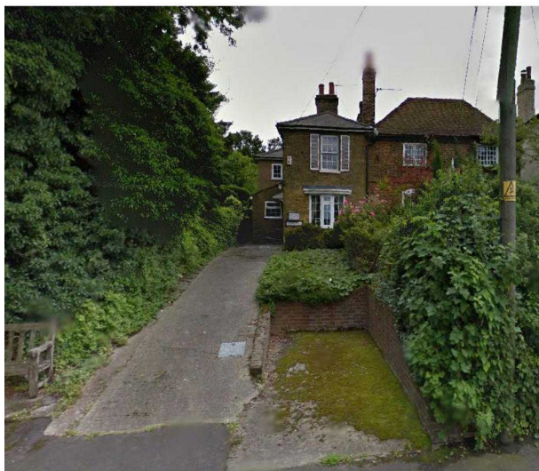
View 4 – Old Pump Cottage in context with Ivy Cottage
