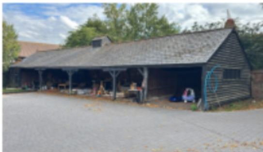
Cart shed and courtyard from the North-west
