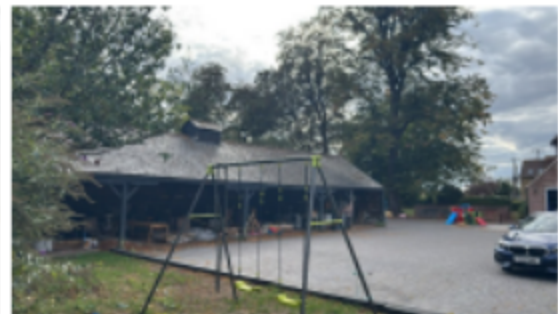
Cart shed and courtyard from the North-east
