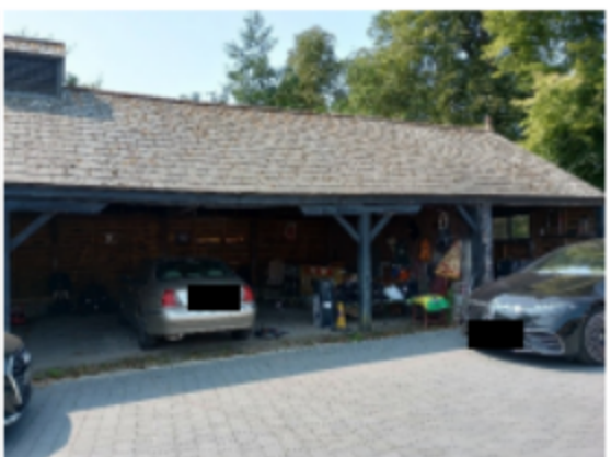
North elevation looking West
