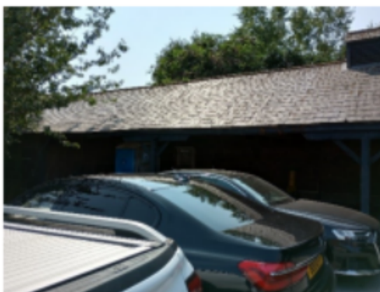
North elevation looking East
