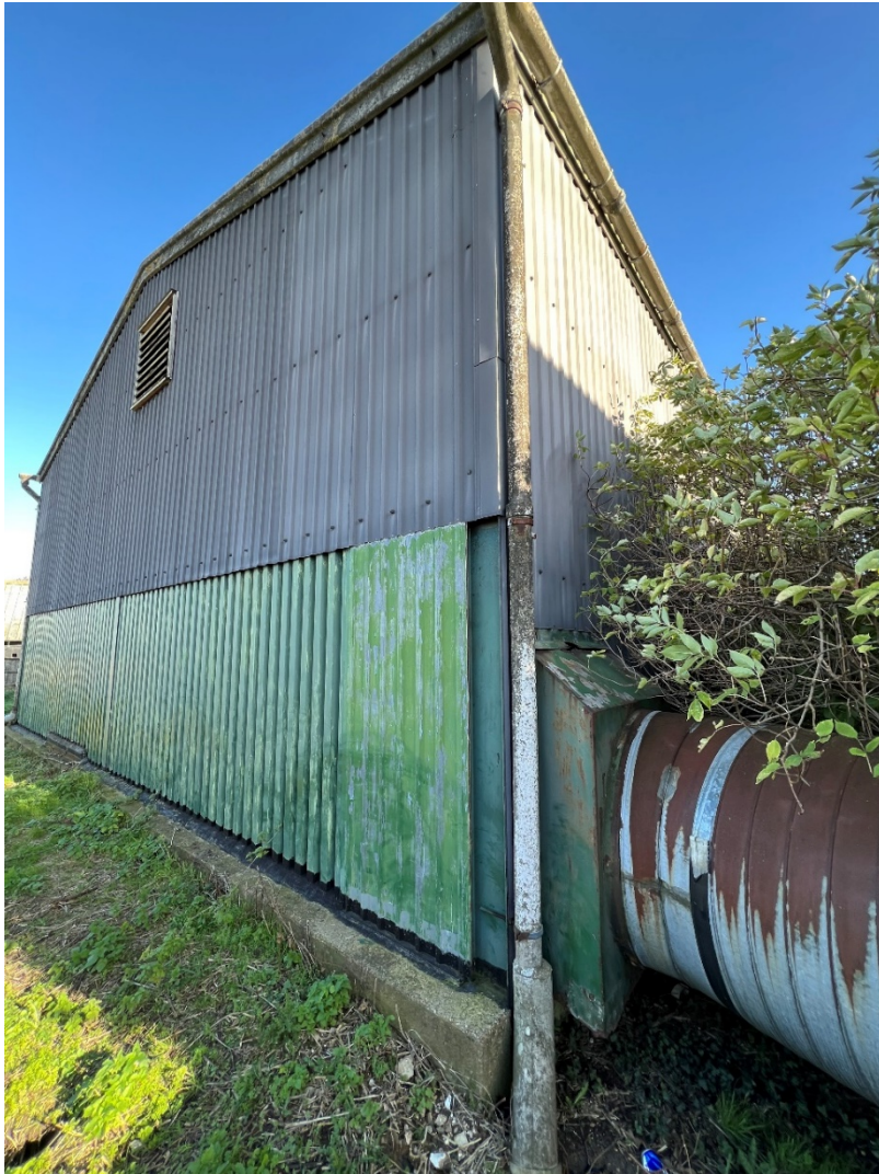
West end of north barn.
