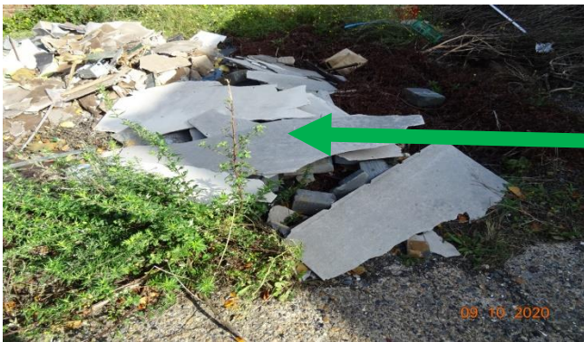
Location Ref 21: Sample TAG/A/S-05- Debris - NO ASBESTOS DETECTED.
