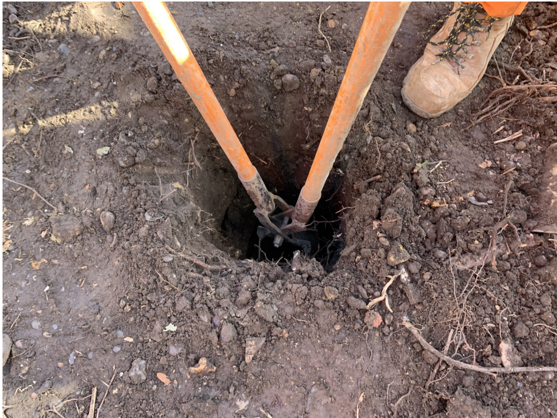
Photo 5: showing hand digging of WS05
