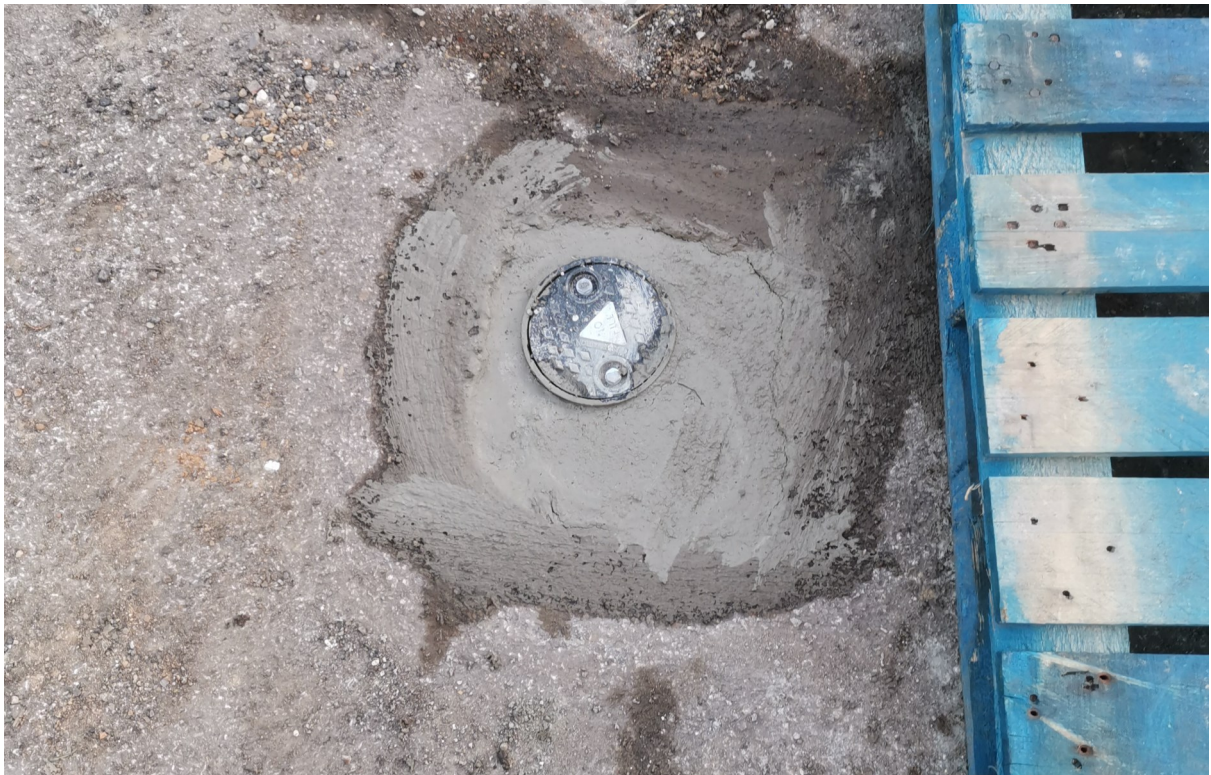
Photo 10: showing WS01 once installed
