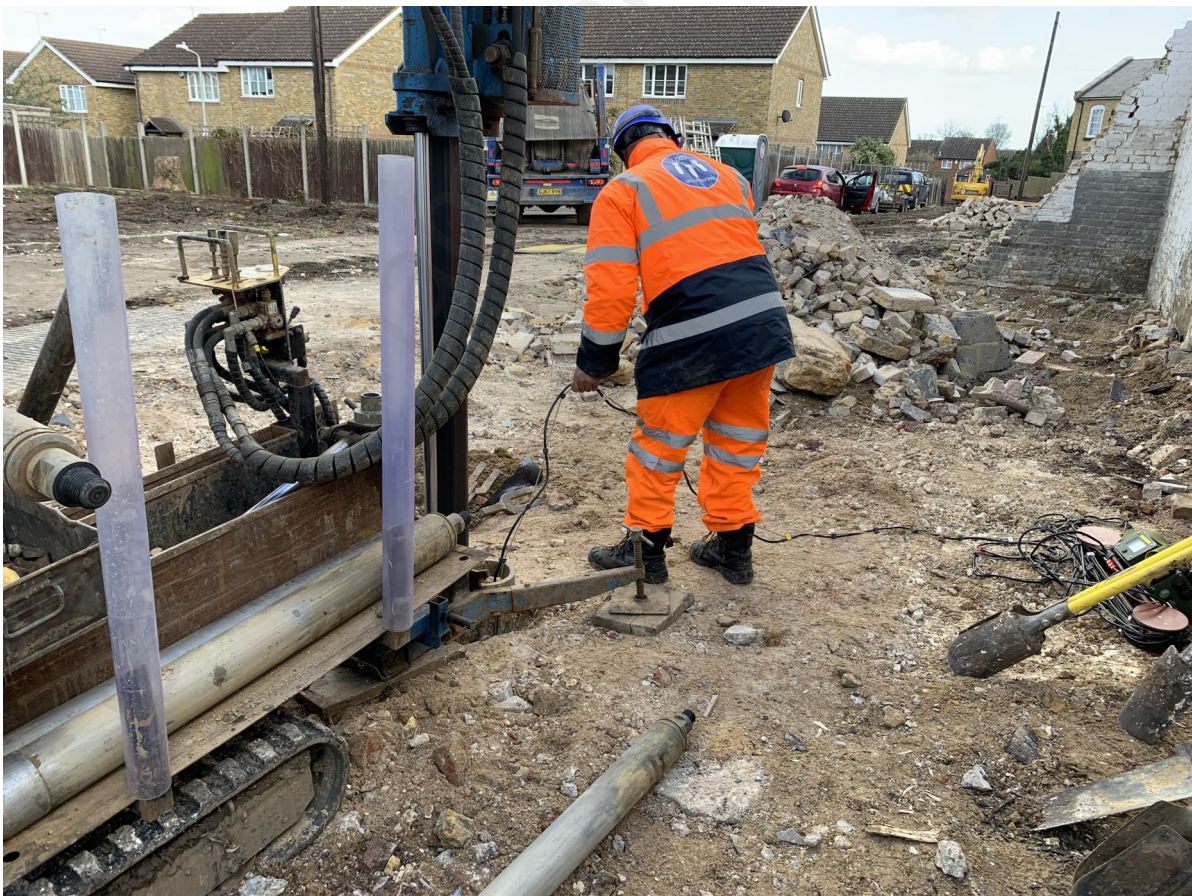
Photo 6: showing WS03 being cleared
