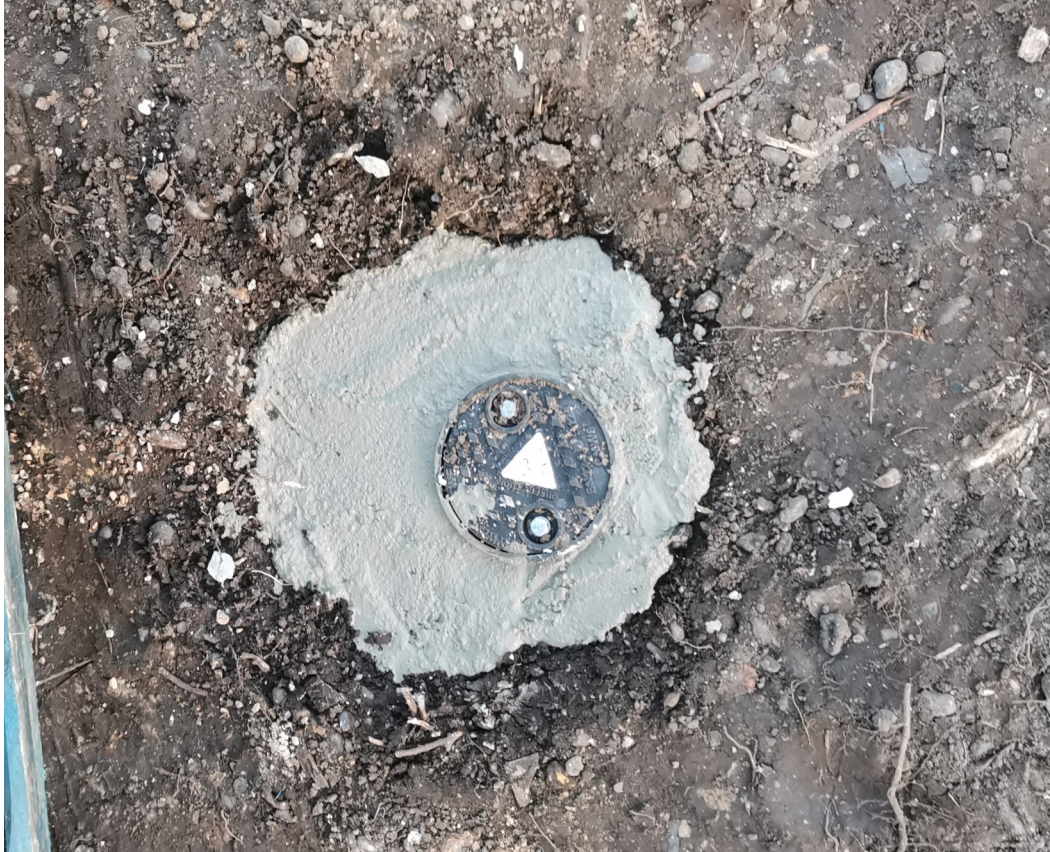
Photo 13: showing WS05 once installed
