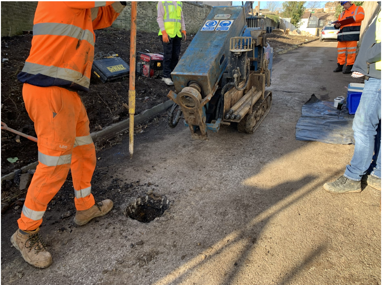
Photo 2: Showing breaking out WS01 position
