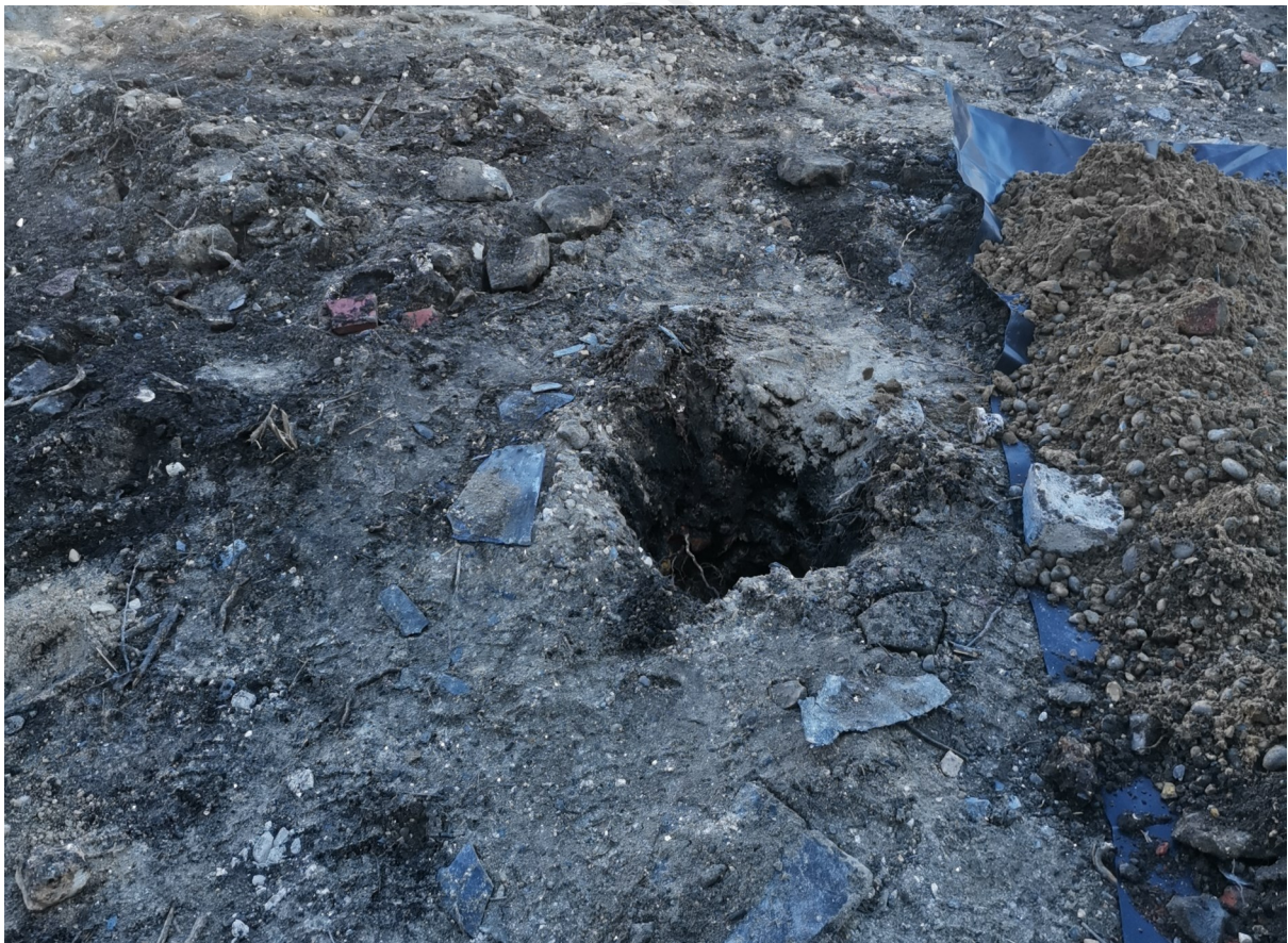
Photo 6: showing TP03 once dug
