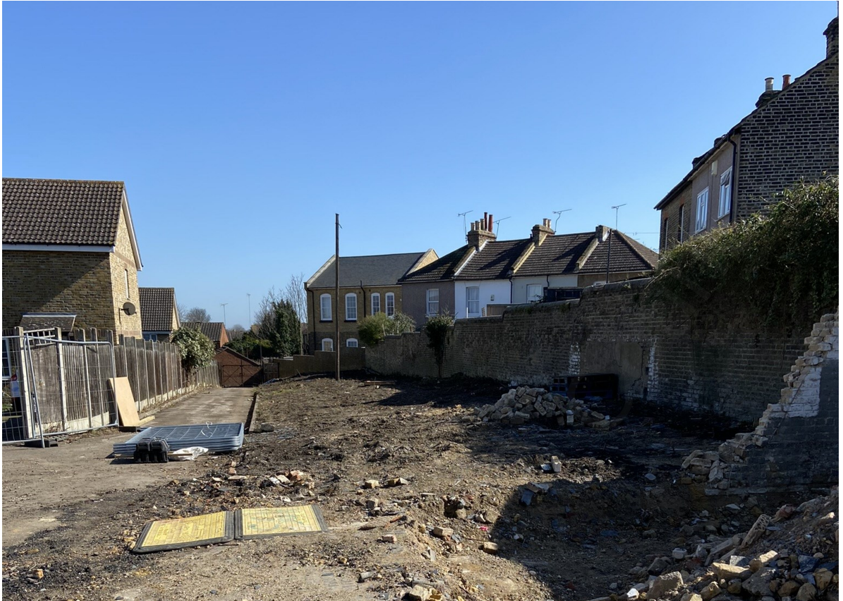
Photo 1: Easterly view down site
