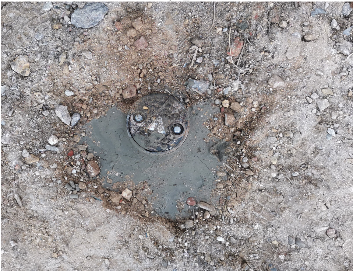
Photo 12: showing WS03 once installed
