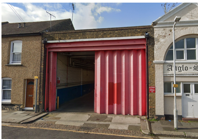
Berkley Road Exit / Entrance.
