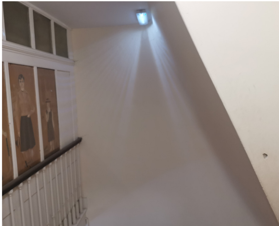
P003 – second floor landing
