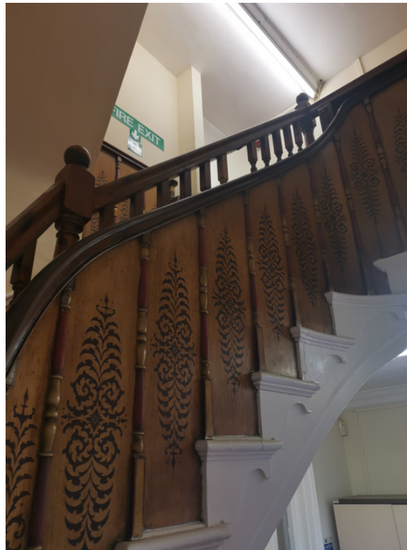
P009 – halfway down second to first stair balustrade detail
