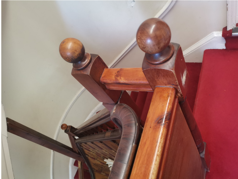
P020 – first floor handrail detail [ note original balustrade and new]
