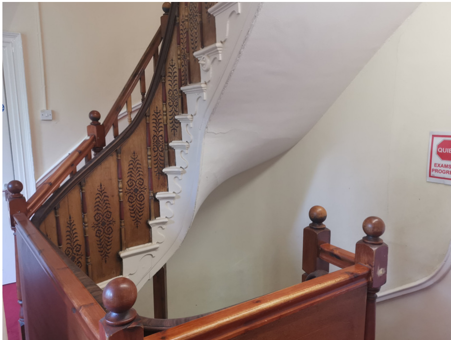
P025 – first floor stair looking down to ground floor
