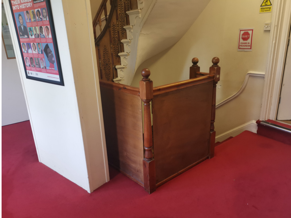
P017 – return landing of first floor stair to ground
