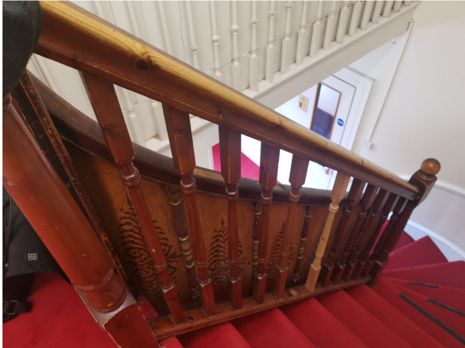
P008 – second floor balustrade detail
