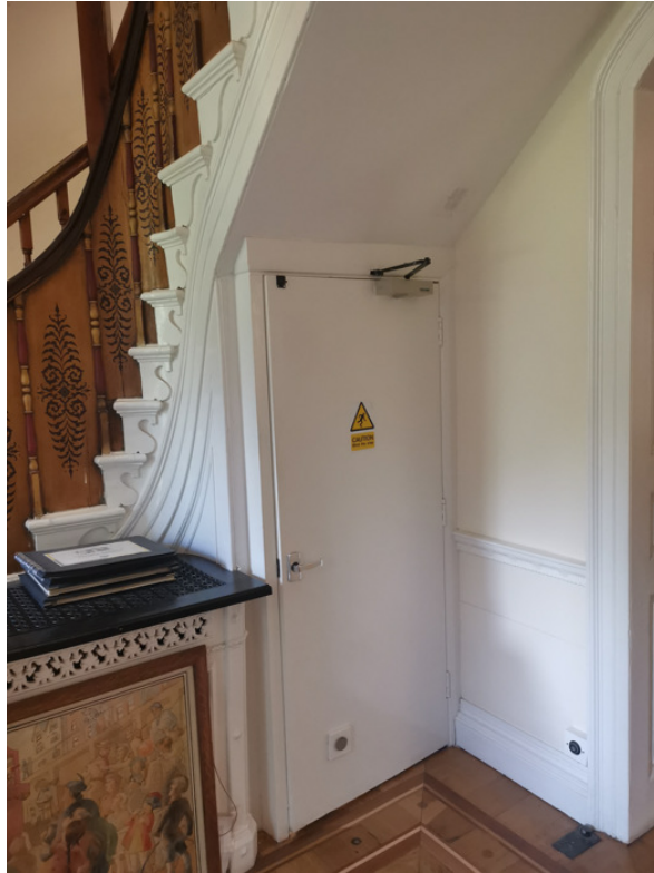
P028 – basement door and heater enclosure
