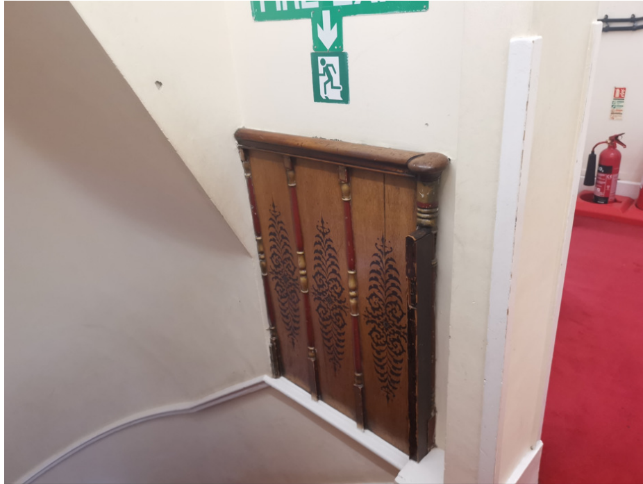
P004 – second floor wall side railing
