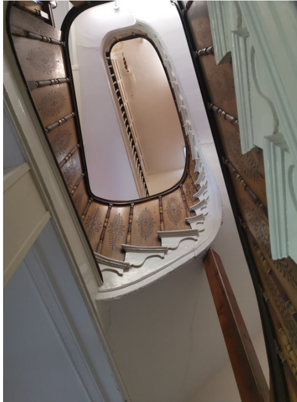
P030 – ground floor looking up thru centre of helical stair
