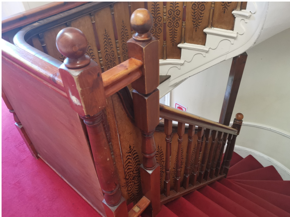
P021 – first floor handrail detail [ note original balustrade and new]
