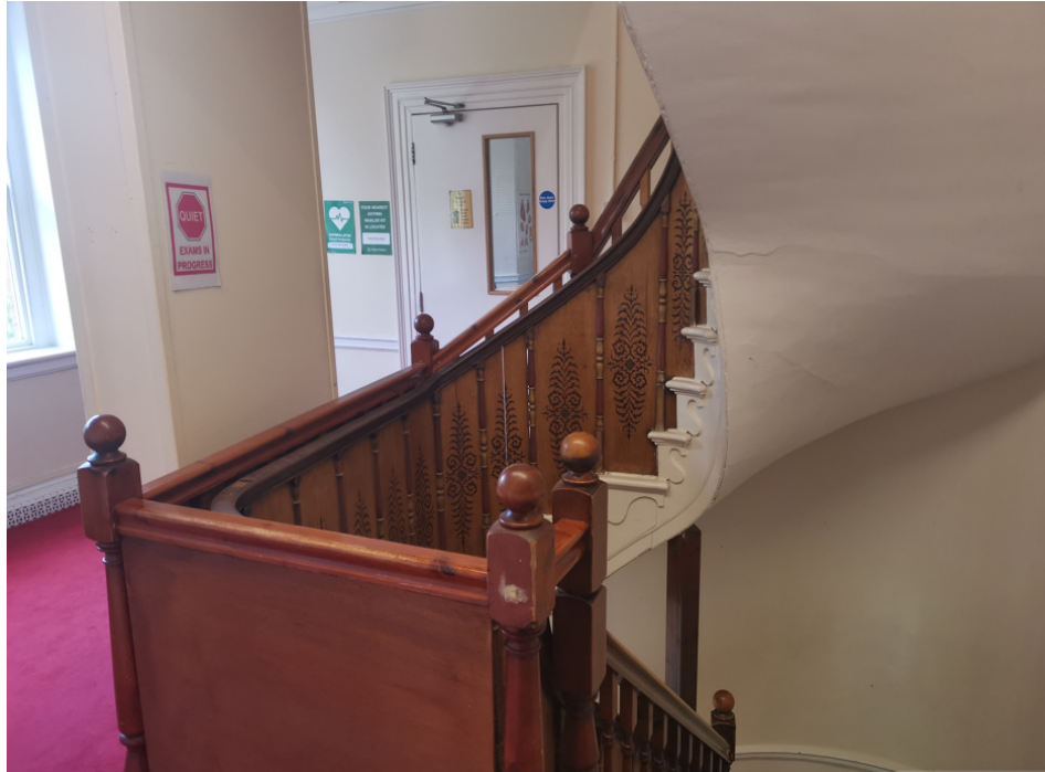
P022 – first floor landing [note area for opening up investigations]
