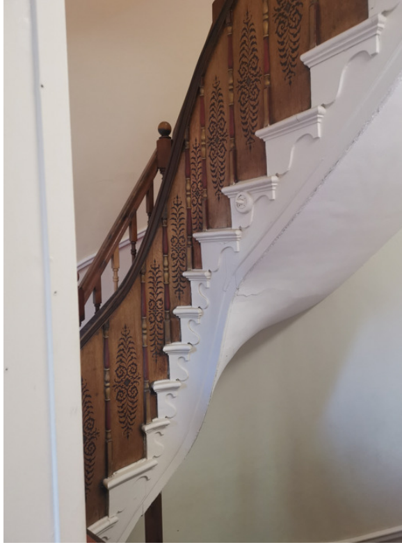
P016 – first floor balustrade detail [note area for opening up investigations]
