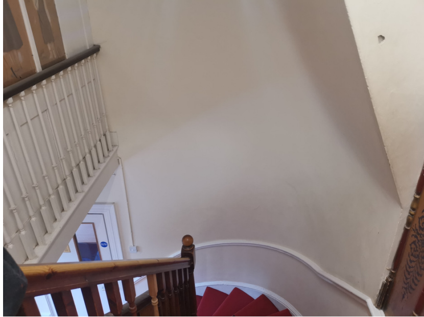
P006 – second floor landing looking down stair
