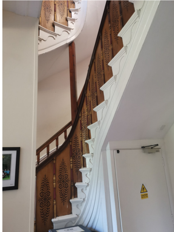
P029 – ground floor stair looking up to first
