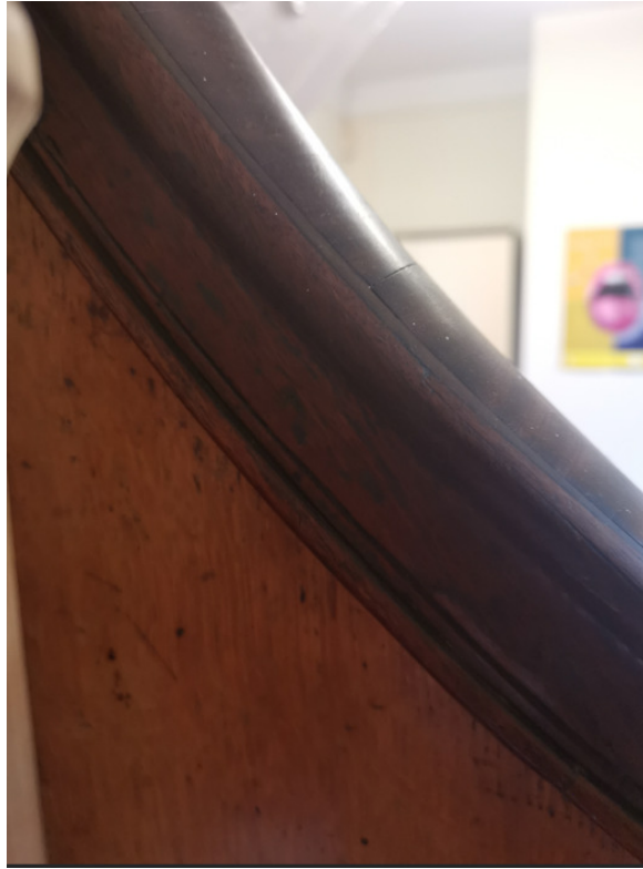
P012 – handrail detail
