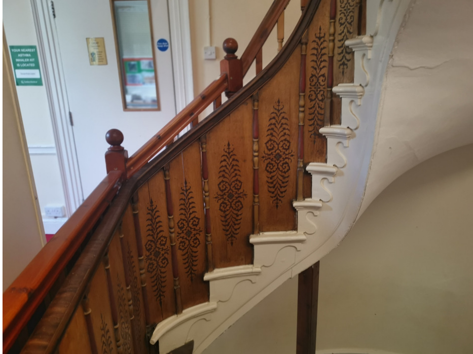
P018 – first floor balustrade detail [note area for opening up investigations]
