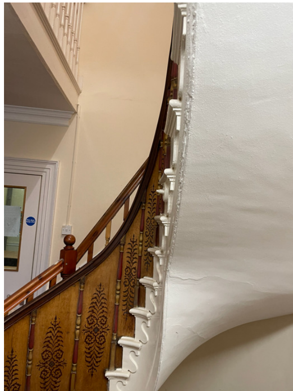
P023 – first floor landing indicating stair under lining [note area for opening up investigations]
