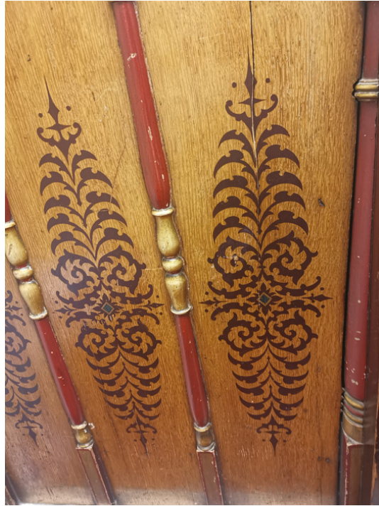
P02 - baluster spindle with hand painted infill [painted stencil by Dickens daughter Kate] alternate balustrade spindle were removed in their place, Dickens had custom fretwork wooden panels inserted. These decorative panels were then beautifully hand-painted by his daughter, Katey (Kate Dickens)
