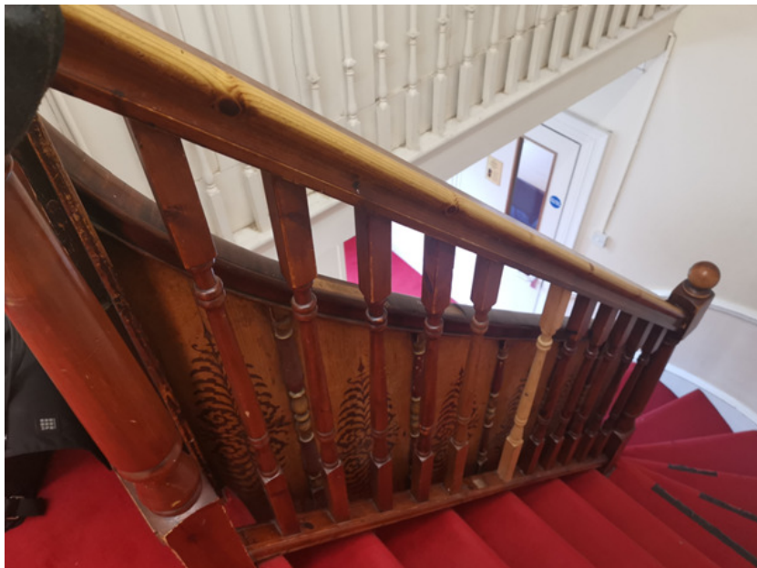
P03 – detail view of original balustrade and protective pine balustrade
