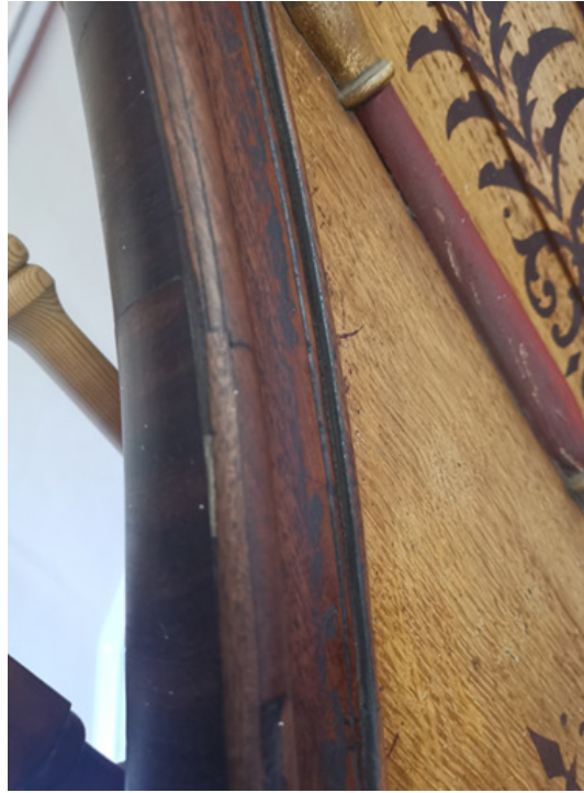
P04 – detail view of original handrail and balustrade
