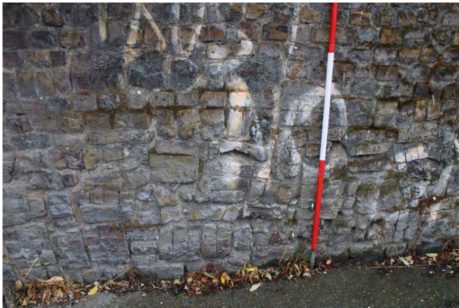
Photo 8: View southeast along the retaining wall of the Site on Athboy Road showing a possible former blocked opening in the wall
