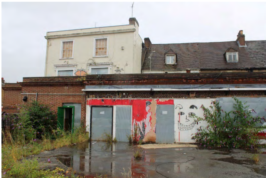
Photo 18: View east across the northeastern half of the Site towards the rear of the Bridge Bar and Club and other properties fronting Stone Street and area of former modern conservatory
