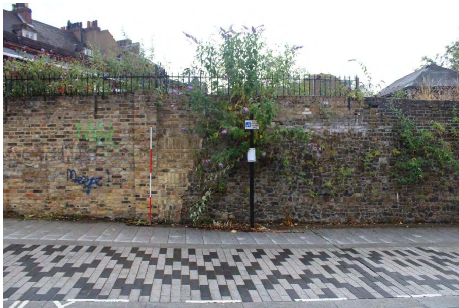
Photo 4: View south along Athboy Road of eastern end of rear garden retaining wall comprised of modern brick to left and rubble stone to right
