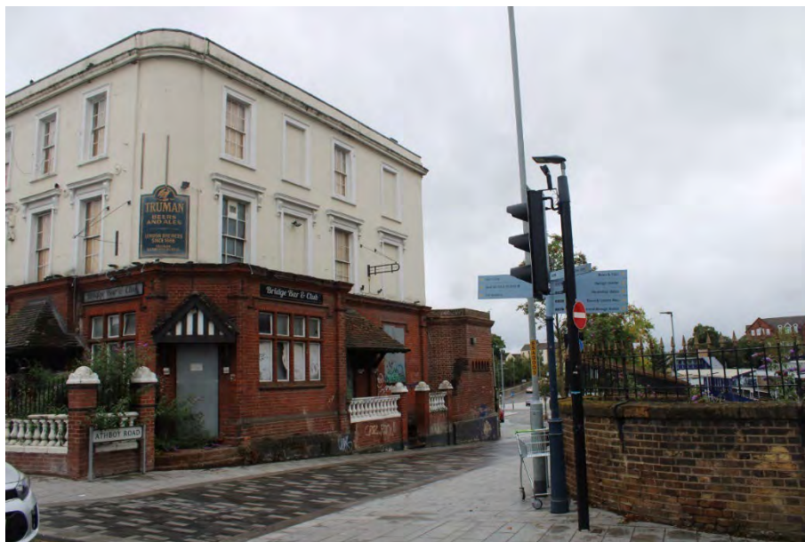
Photo 2: View southwest of the Bridge Bar and Club looking along Athboy Road
