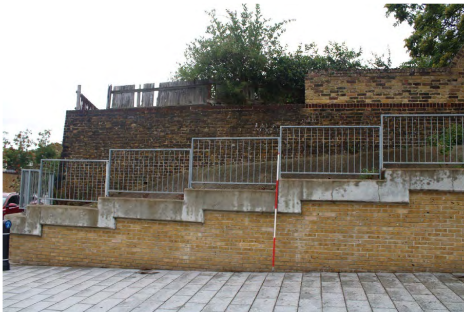
Photo 11: Northern end of western retaining wall along the Site between Athboy Road and the A 226
