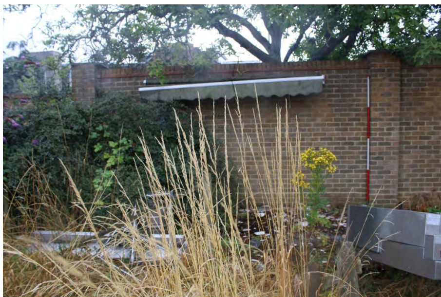
Photo 35: Modern brick built garden partition wall on western side of Site, looking towards the south
