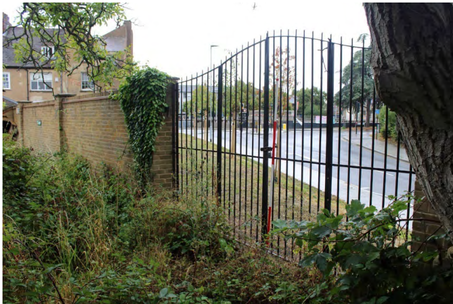
Photo 24: View southeast along southern boundary wall and former entrance gateway looking towards junction of A226 and Stone Street
