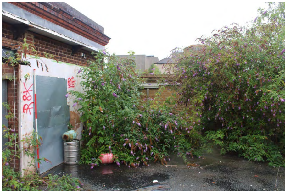
Photo 20: View of southeastern corner of the Site, showing part of southern boundary wall and small brick built shed
