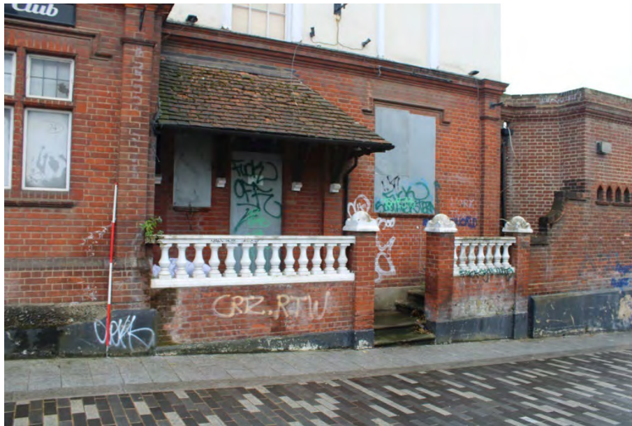
Photo 3: View southwest of the eastern end of the Bridge Bar and Club and the start of the rear yard area (modern brick walling to right) from Athboy Road
