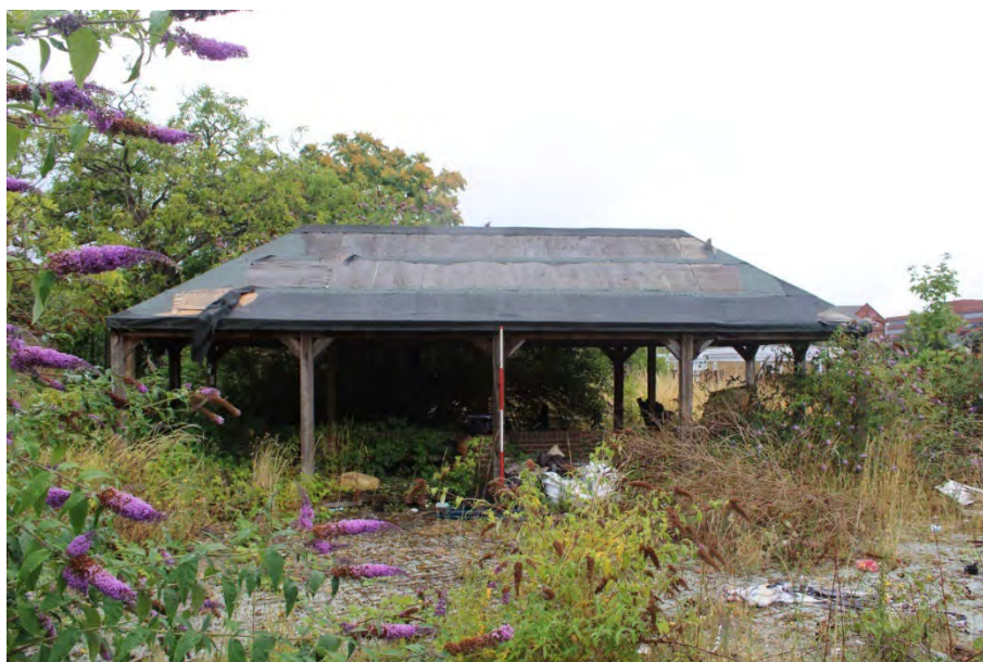
Photo 28: View west of the modern timber gazebo in the centre of the Site
