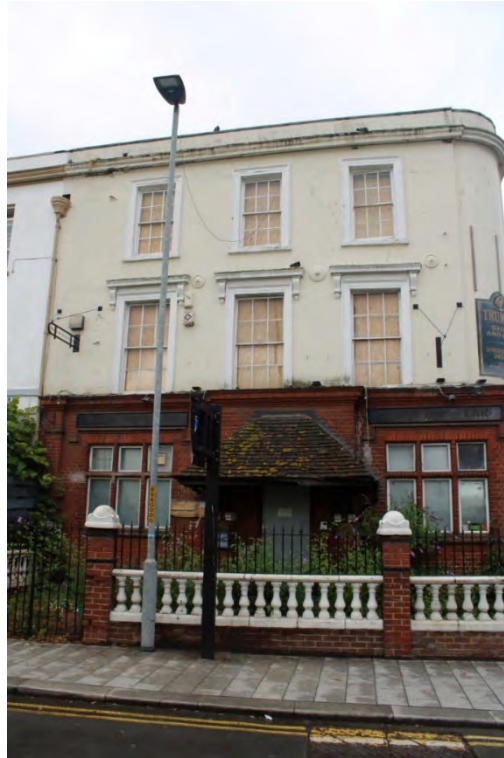
Photo 1: View west of the Stone Street façade of the Bridge Bar and Club
