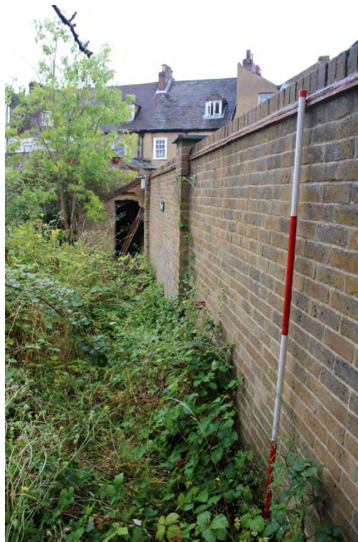
Photo 22: View east along southern boundary wall of the Site towards the brick built shed and the rear of properties fronting Stone Street
