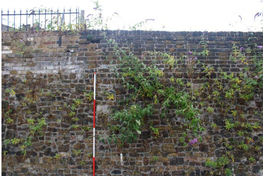
Photo 5: View south along Athboy Road of eastern half of retaining wall around the Site showing change in top of wall from modern brick and metal railings to older dark bricks
