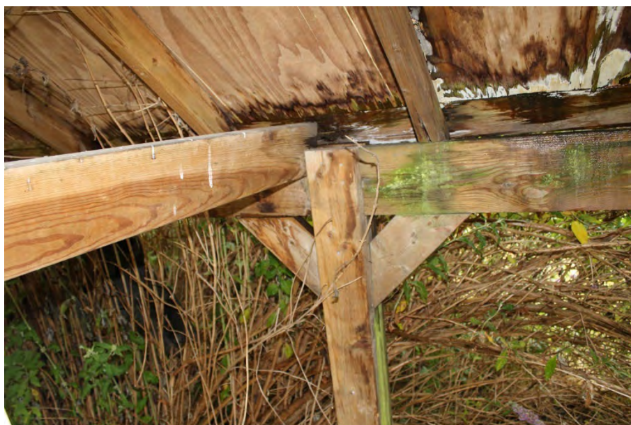
Photo 31: Detail of timber upright joint with roof of the modern timber gazebo
