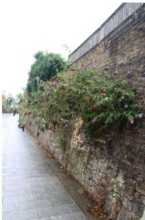
Photo 10: View east along retaining wall of Site along Athboy Road
