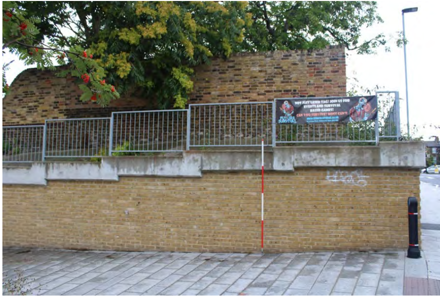
Photo 13: View of western retaining wall around the Site at its southern end, with A226 to right
