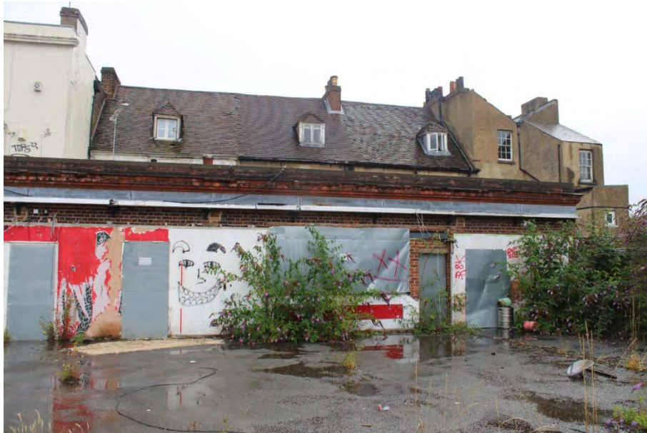
Photo 19: View east across the southeastern half of the Site towards the rear of properties fronting Stone Street and area of former modern conservatory
