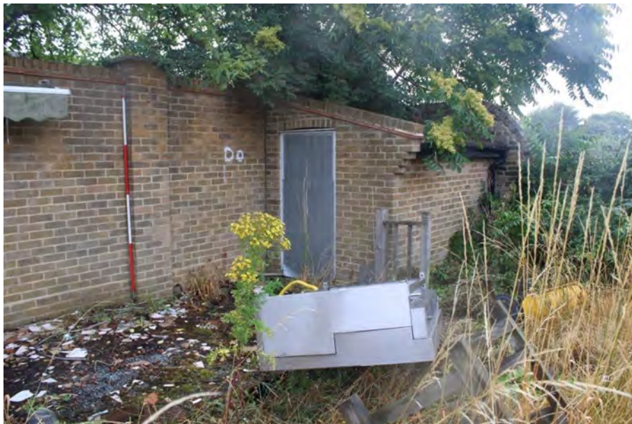
Photo 34: Modern brick built garden partition wall on western side of Site, including small shed or toilet, looking towards the western end wall
