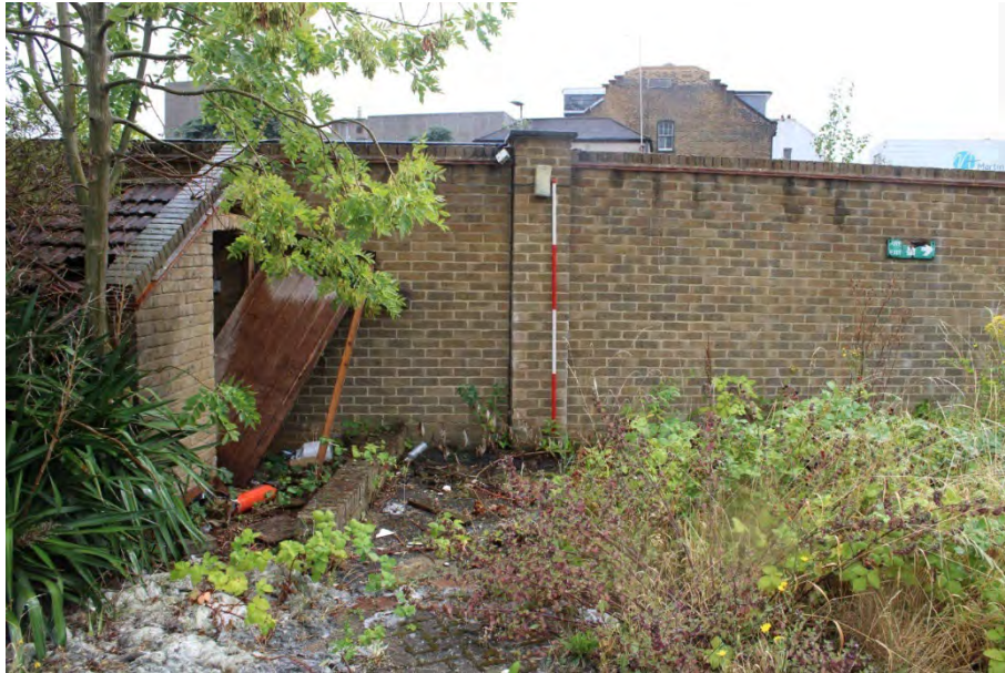
Photo 21: View of the southern boundary wall around the Site, with brick built shed to left
