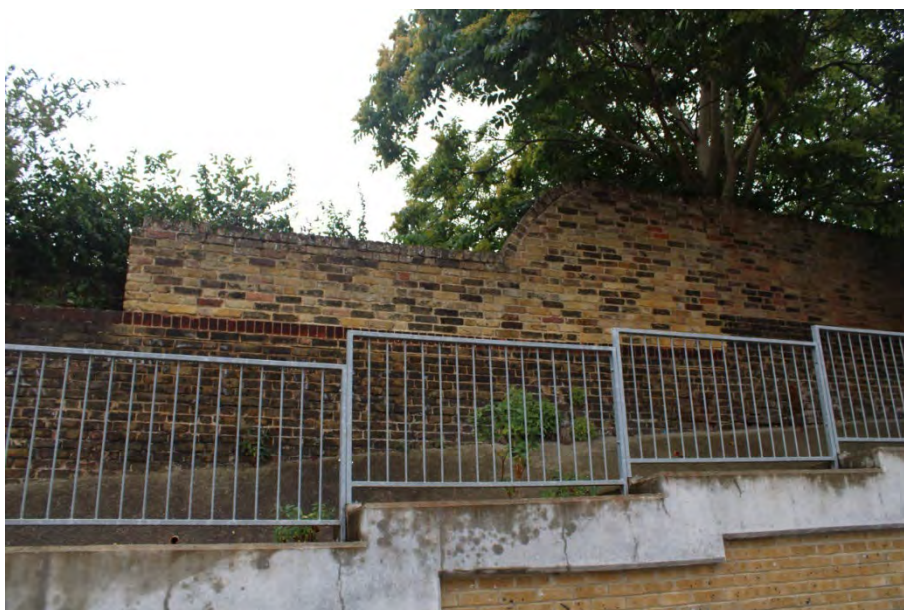
Photo 12: View of central part of the western retaining wall around the Site
