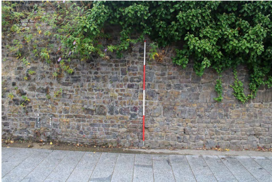
Photo 7: View along Athboy Road of western side of retaining wall of Site showing different construction phases and elements of patching in the walling
