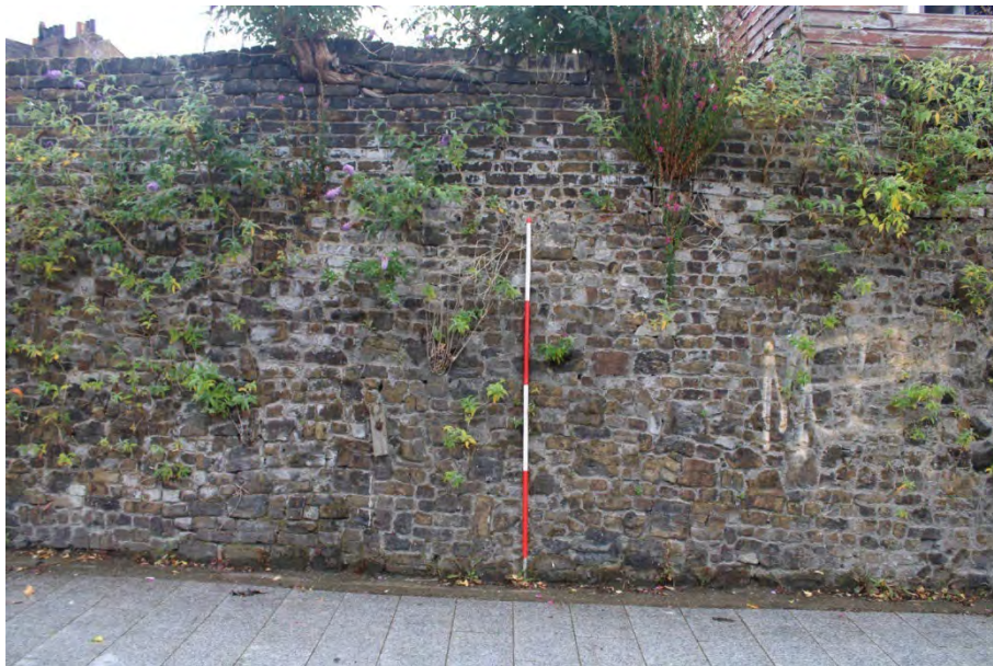
Photo 6: View along Athboy Road of centre of retaining wall of Site showing different construction phases
