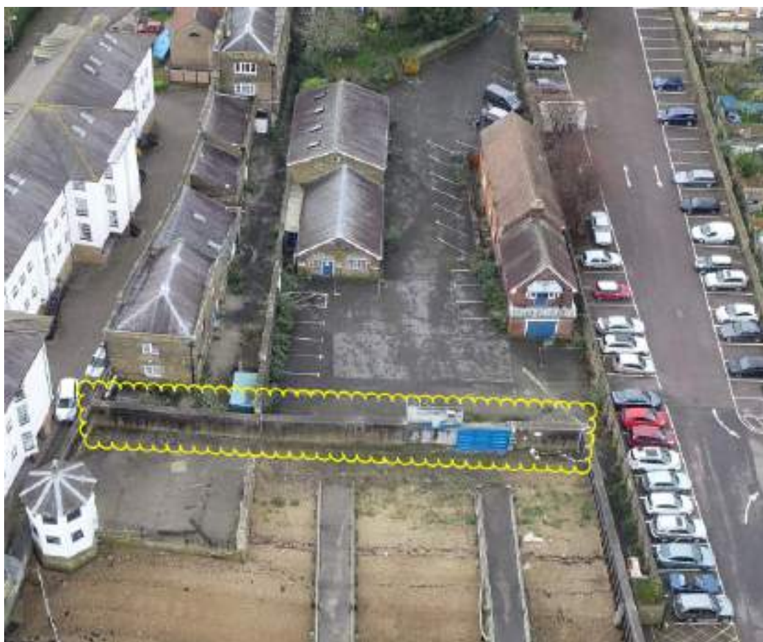
Photograph 2.0 - Existing steel sheet piled wall, encased in concrete and clad in masonry
