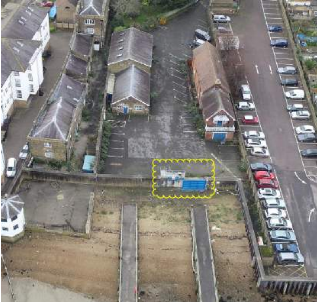
Photograph 3.0 Flood gate and stair location
