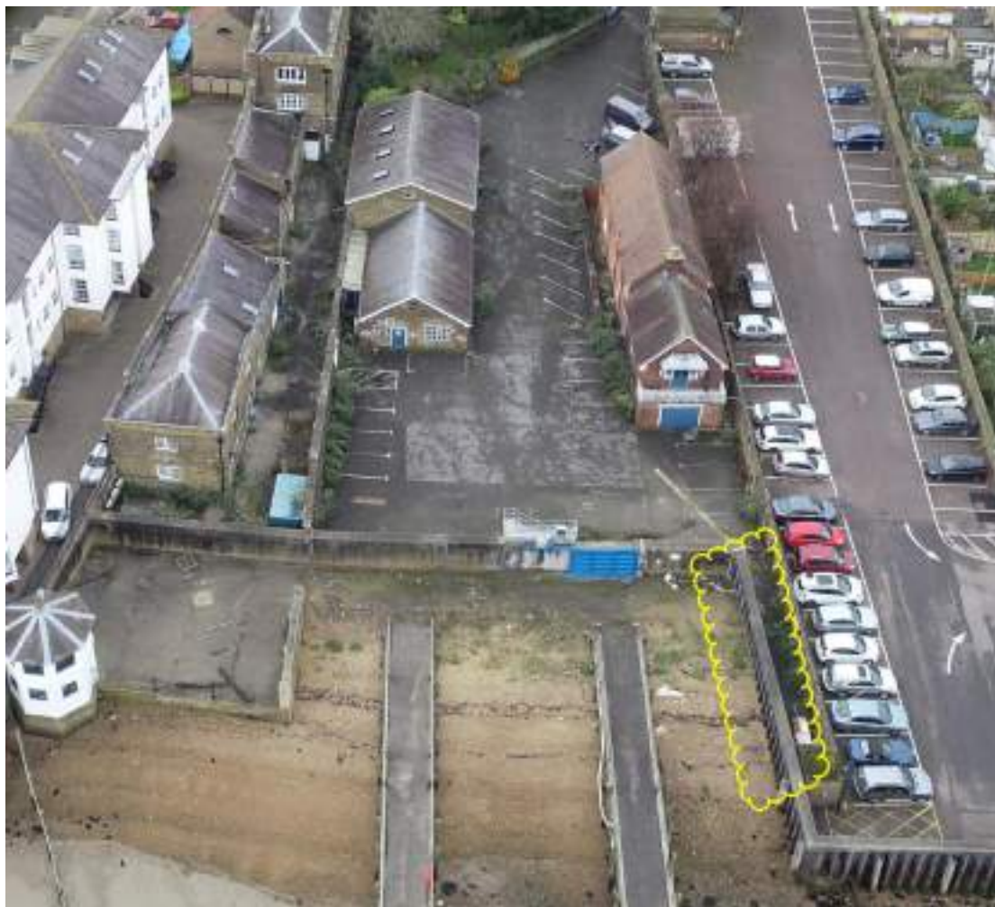
Photograph 1.0 - The length of existing exposed steel sheet piled wall
