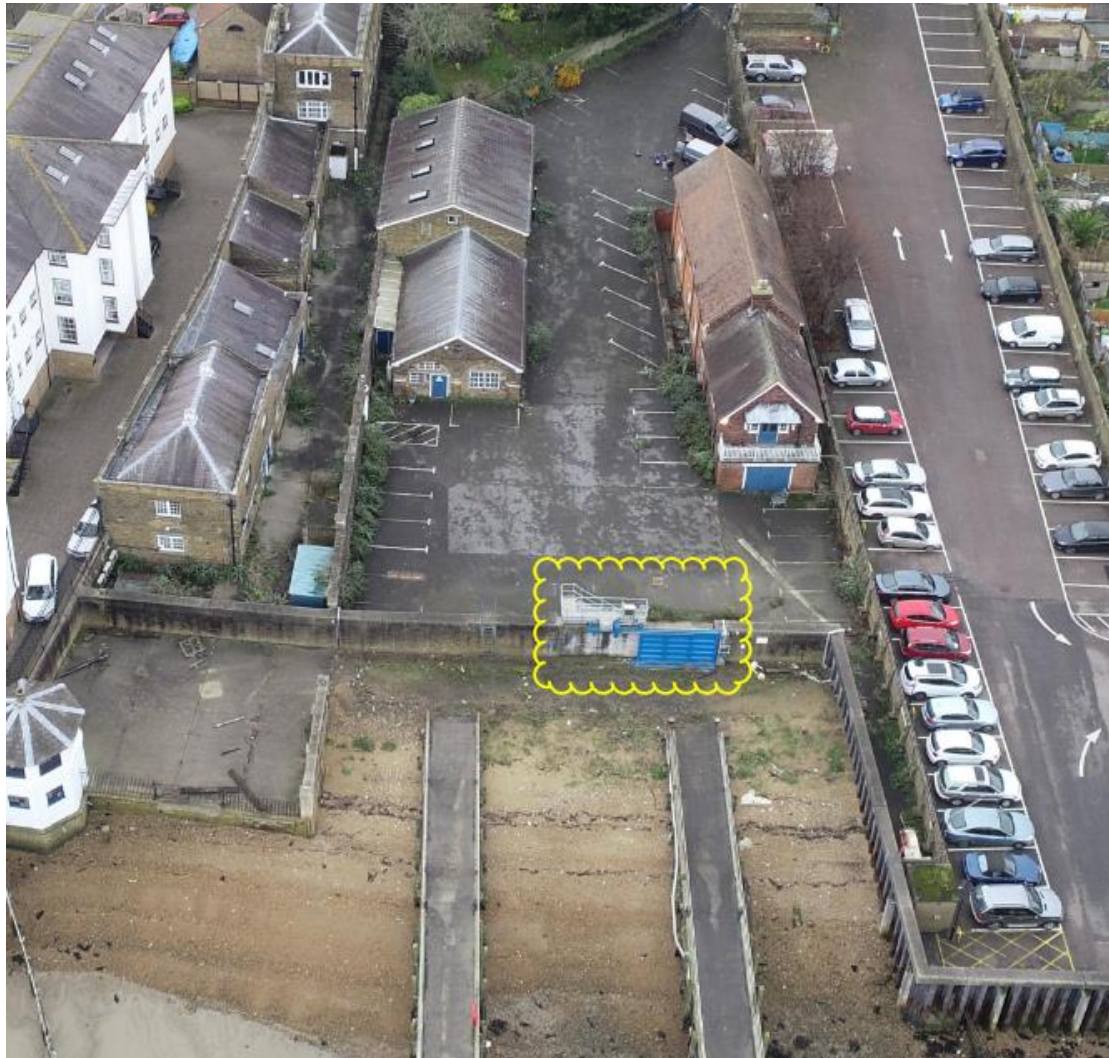
Photograph 3.0 Flood gate and stair location
