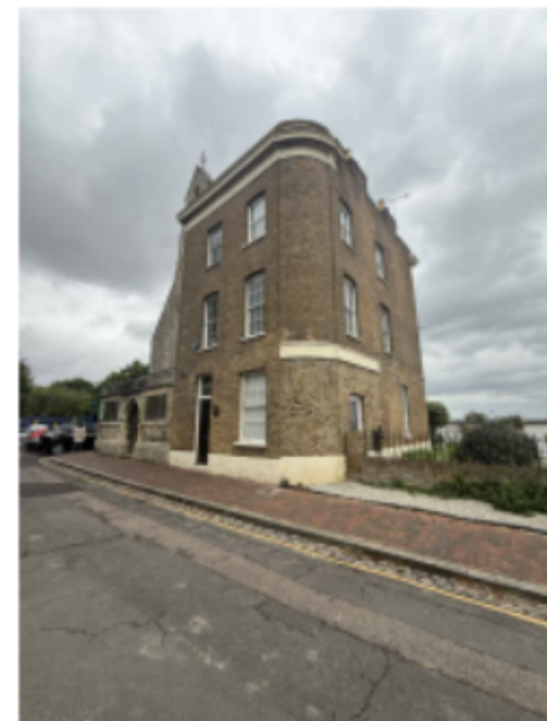
VIEW OF ST ANDREWS/MISSION HOUSE FROM THE EAST
