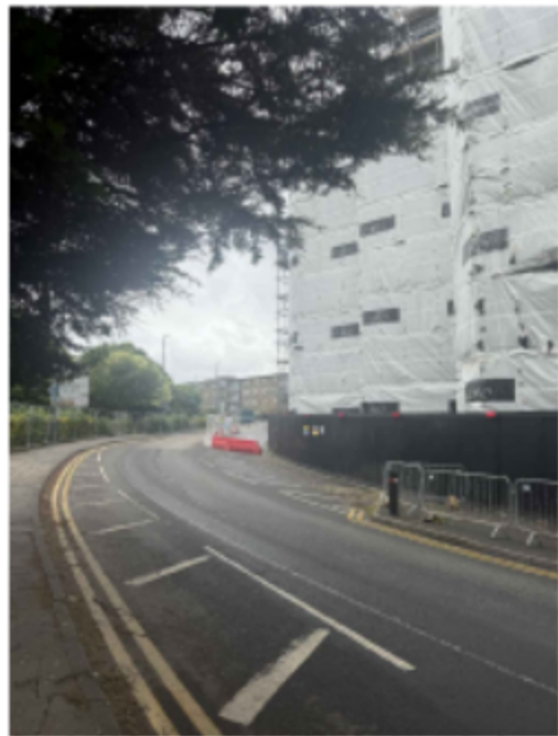
BUILDINGS UNDER CONSTRUCTION ALONG THE SOUTH SIDE OF CROOKED LANE
