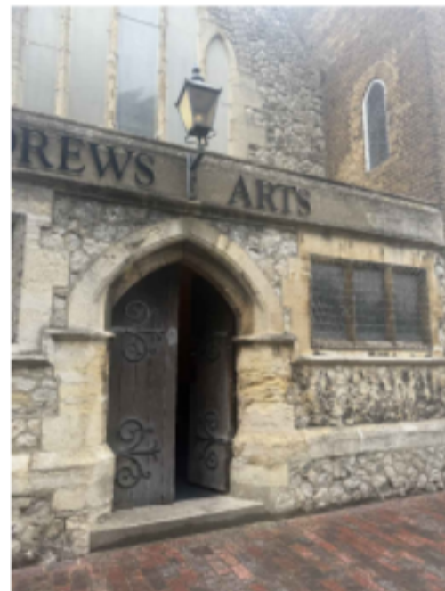
ST ANDREWS' FRONT ENTRY
