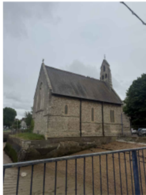
VIEW FROM WATERFRONT LOOKING TOWARDS REAR OF ST ANDREWS'
