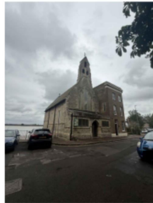
ST ANDREWS' AND THE ADJOINING MISSION HOUSE BUILDING
