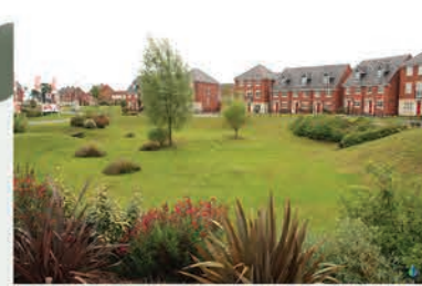
SuDS attenuation basins and swale features with planting which is tolerant of both wet and dry conditions; Close mown path with seating around the SuDS attenuation basins
