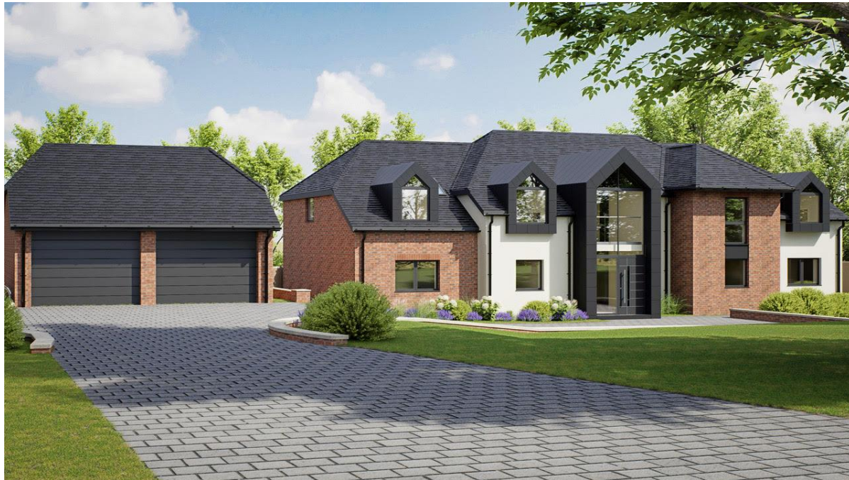
View at entrance
