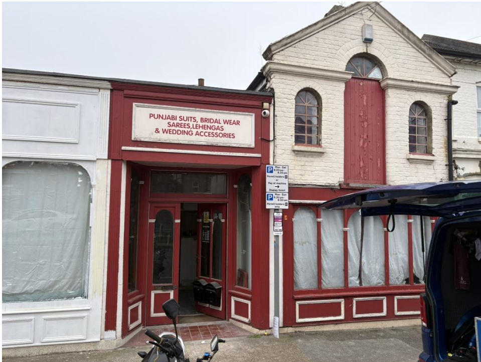
Figure 7- Existing front of the building.
