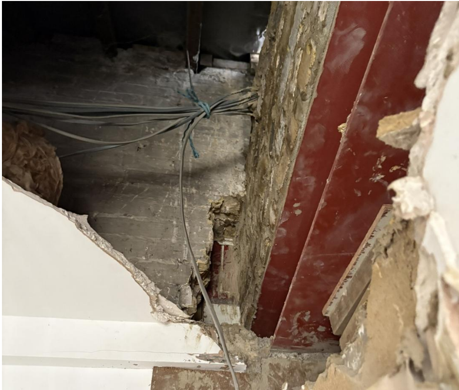
Figure 5- Structural beam installed into separating wall. Ensure any gaps are adequately sealed.
