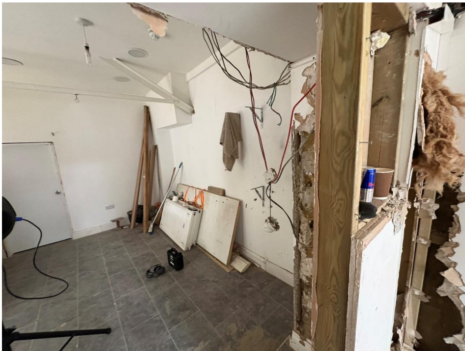
Figure 6 – Current separating wall condition during site visit and test.
