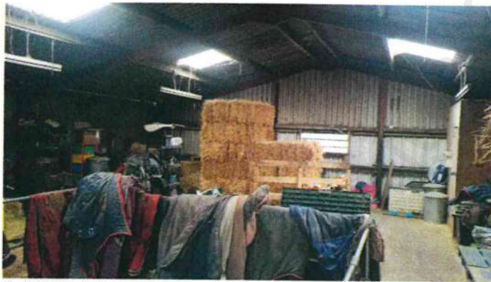
5. Internal above mezzanine level.
