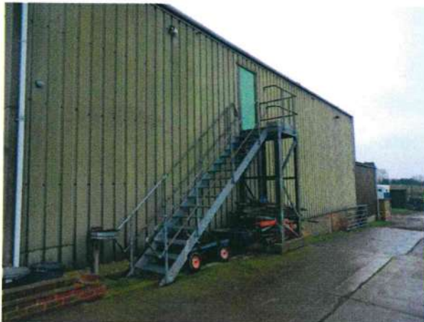
4. Right elevation and access stair
