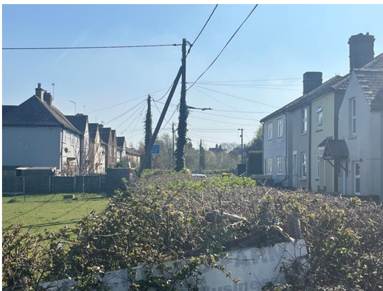
Plate 18: Eastwards view of the rooftop of Dairy Farmhouse from the roadside entrance into the site off Chalk Road.
