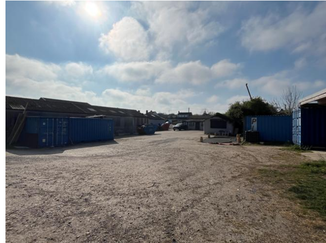
Plate 3: The existing built form and courtyards within the site.
