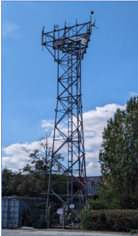
Figure 2: Existing tower at Denton Wharf
