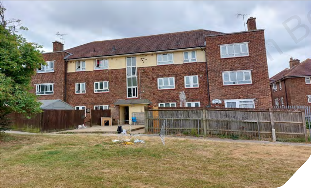
Plate 03: North-eastern Three-storey Building Block
