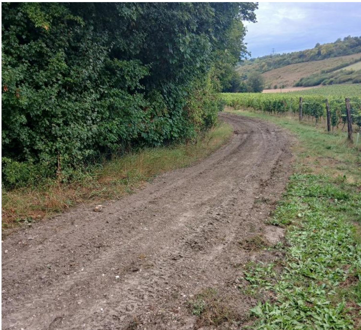
Figure 2: Typical image of farm track at Luddesdown Road
