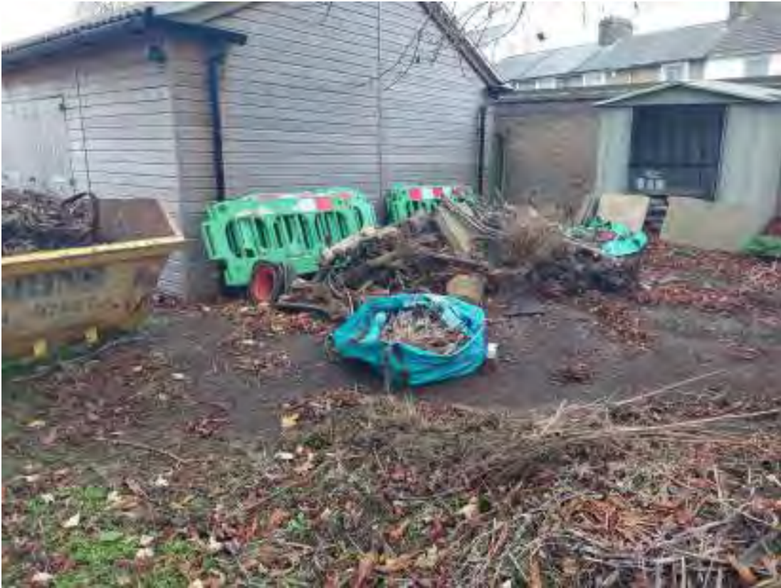
Photo 11—skip comprising rubble and organic matter such as bark, soil and wood. Barriers and cones, and a stockpile of wood, bark, and soil was noted adjacent to the skip
