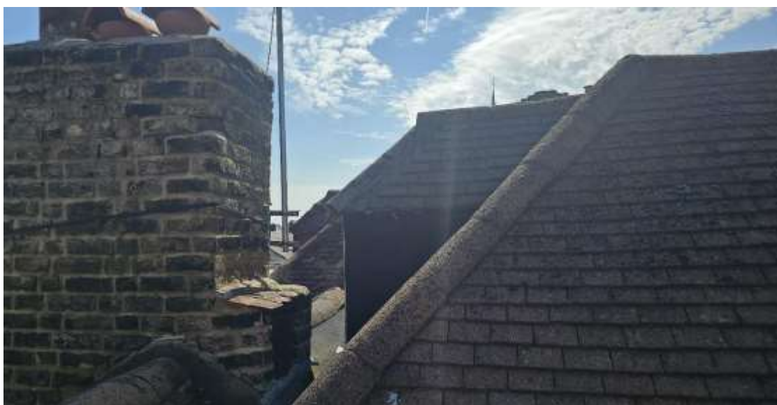
Fig.11: Existing rear dormer and chimney of no.3.
