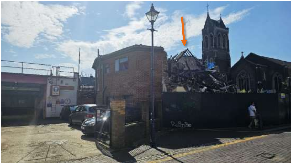
Fig.4: View southeast from Queen Street.
