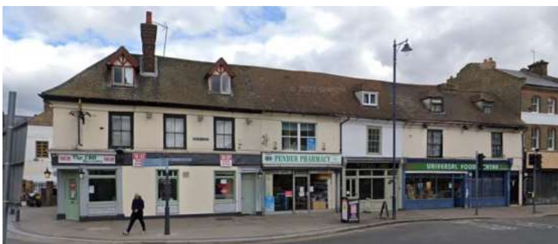
Fig.12: Nos.1-5 Milton Road in 2021, prior to the fire.
