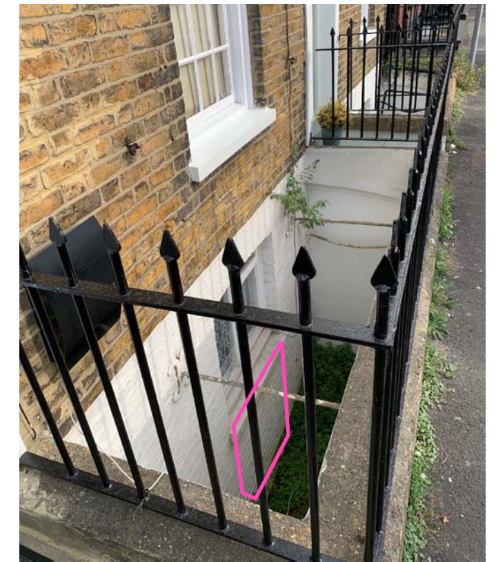
Portion of brickwork to be removed
