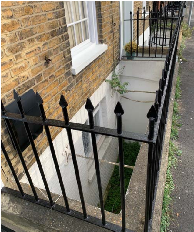
View of the existing lightwell
