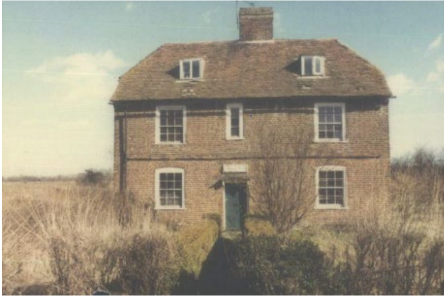
Figure 1 Front Elevation with exposed box sash windows
