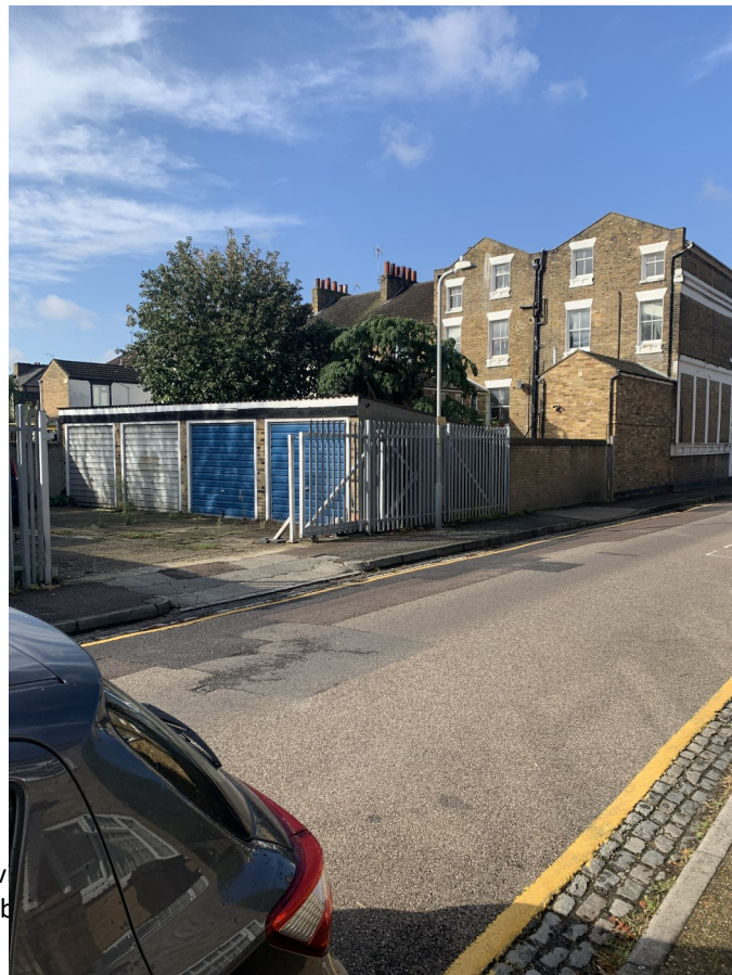
View of existing garages
