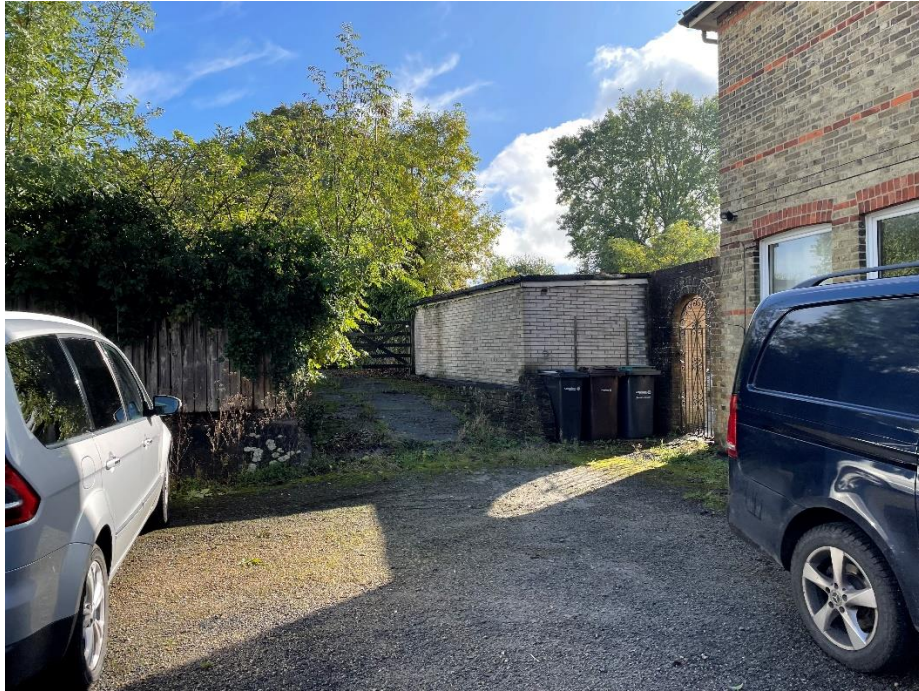
Existing garage / outbuilding to be demolished
