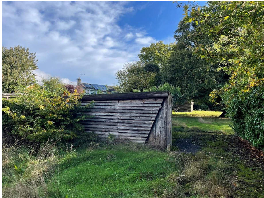
Existing outbuilding to be demolished
