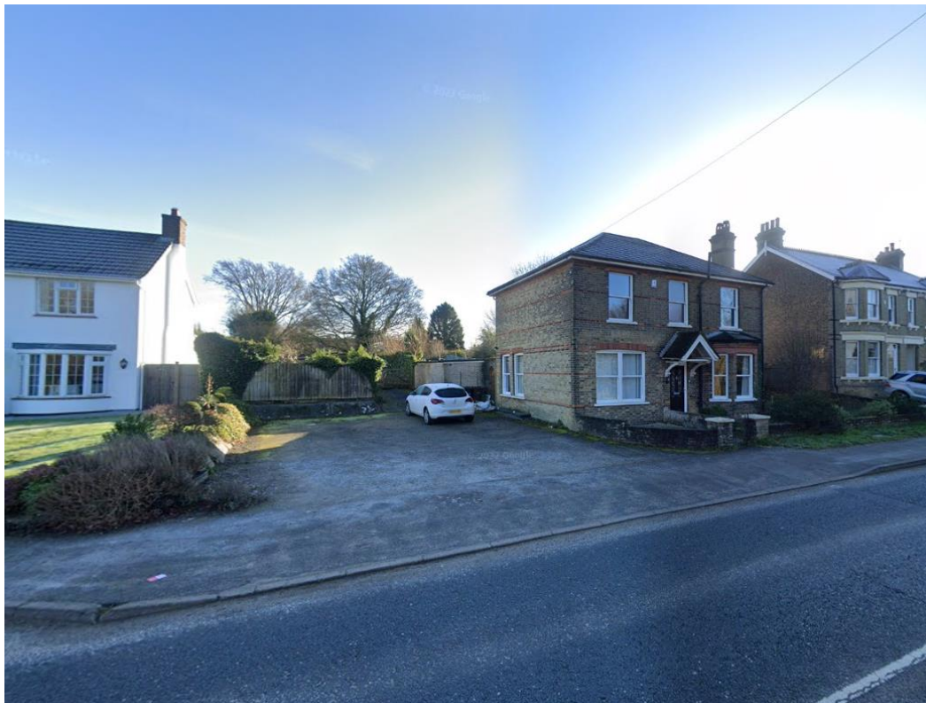
Fig 2 – The site (Northfield House) viewed from Wrotham Road
