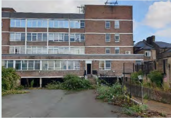
Rear façade of building
