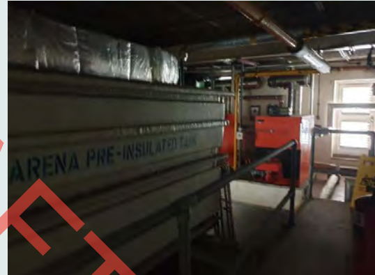
Plant room on roof
