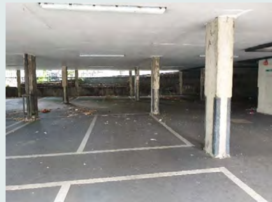
Underground car park
