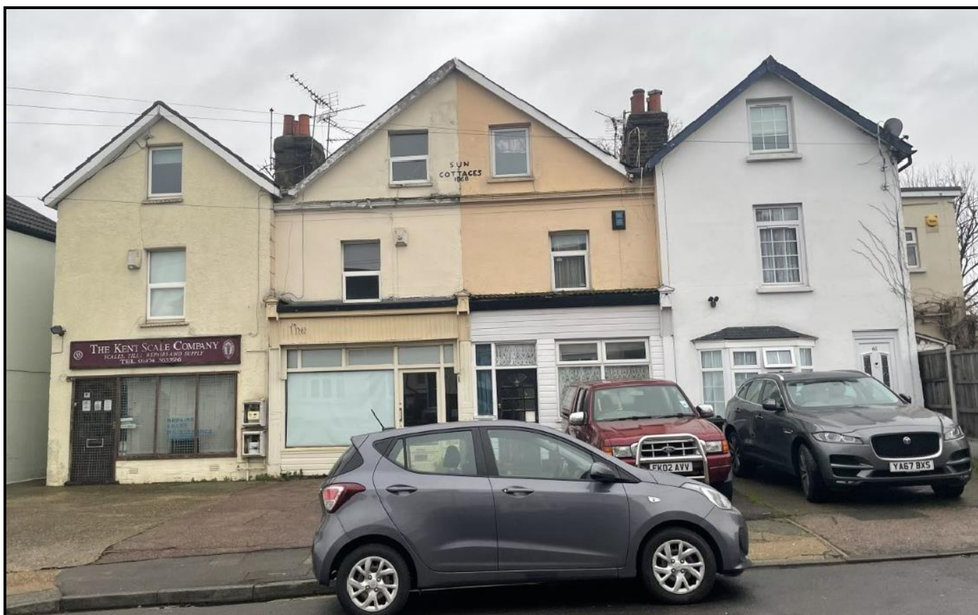
Image of Front Elevation of row of terraced buildings.
