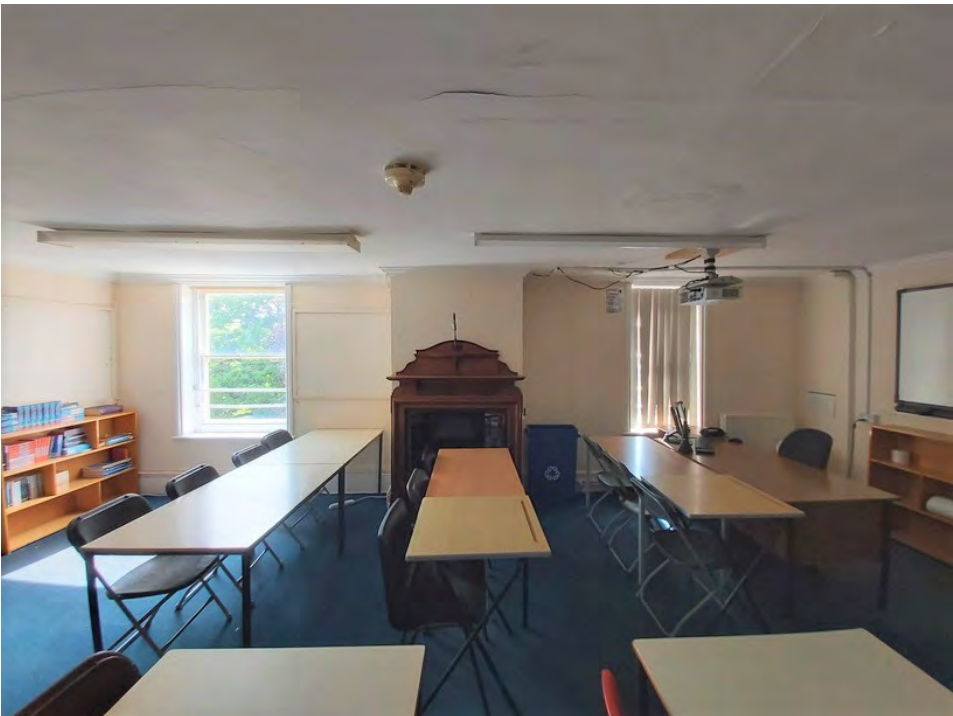
1) Ceiling of HSFX06 H1 classroom looking east Photograph taken 01/08/2022 by CP
