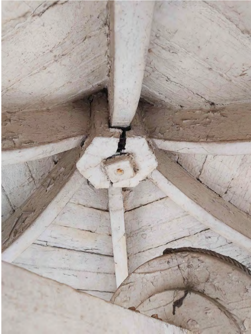
3) Underside of cupola HCPX01. Photograph taken 17/08/2023 by CP
