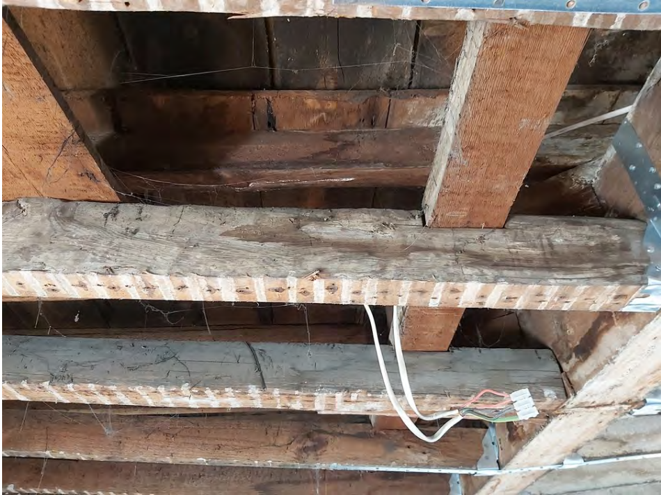
1) Ceiling of HSF06 H1 classroom looking north Underside of lead roof RFX03. Photograph taken 23/11/2022 by CP
