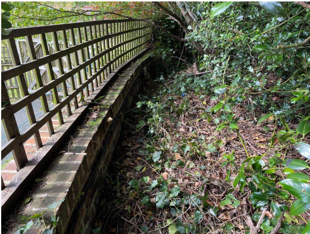
View along top of wall showing proximity of trees and undergrowth
