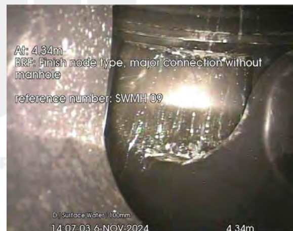
50.jpg, 00:00:29, 4.34 m Finish node, major connection without manhole, reference: SWMH 09
