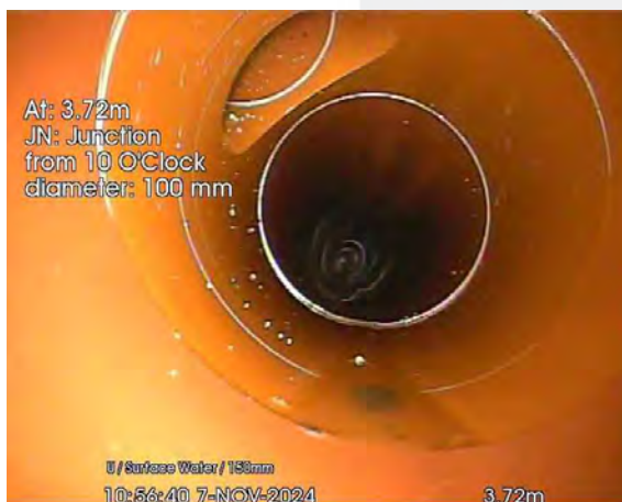
200.jpg, 00:00:17, 3.72 m Junction at 10 o'clock, diameter: 100mm
