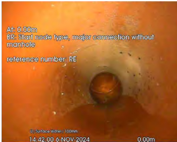
92.jpg, 00:00:01, 0.00 m Start node, major connection without manhole, reference: RE
