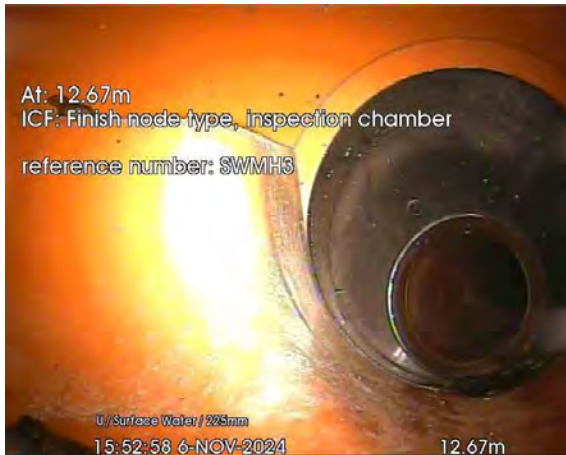
143.jpg, 00:00:29, 12.67 m Finish node, inspection chamber, reference: SWMH3
