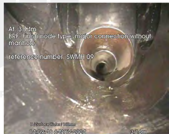
54.jpg, 00:00:22, 3.16 m Finish node, major connection without manhole, reference: SWMH 09
