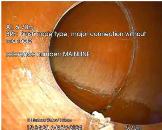
117.jpg, 00:00:24, 5.70 m Finish node, major connection without manhole, reference: MAINLINE
