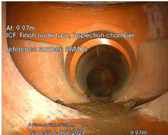
130.jpg, 00:00:37, 9.97 m Finish node, inspection chamber, reference: SWMH6
