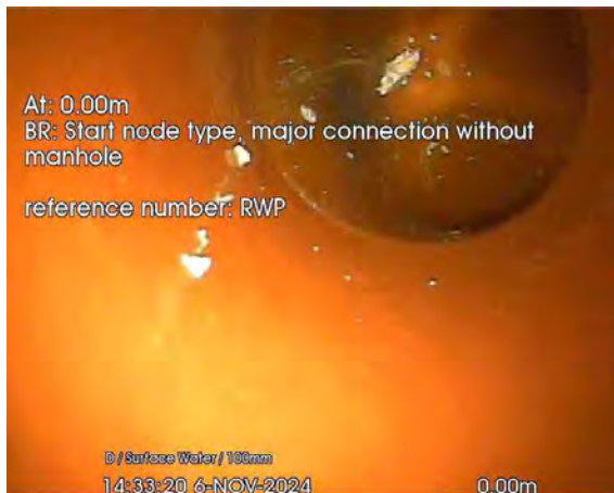
80.jpg, 00:00:01, 0.00 m Start node, major connection without manhole, reference: RWP
