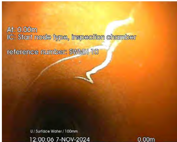
255.jpg, 00:00:02, 0.00 m Start node, inspection chamber, reference: SWMH 10
