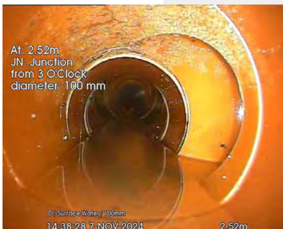
337.jpg, 00:00:23, 2.52 m Junction at 3 o'clock, diameter: 100mm
