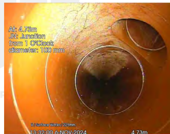
13.jpg, 00:00:29, 4.73 m Junction at 1 o'clock, diameter: 100mm
