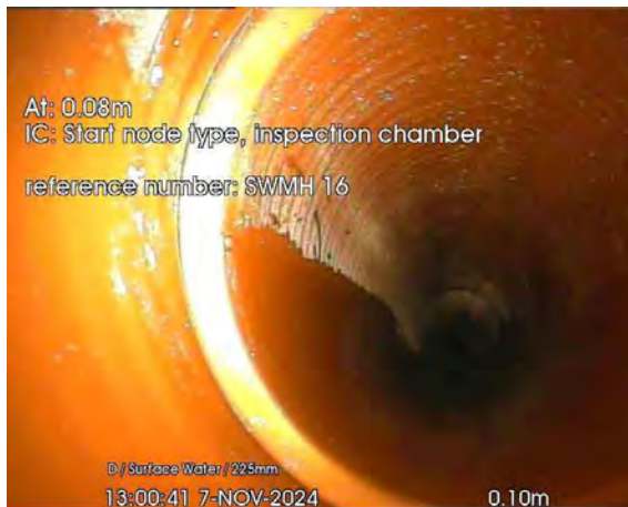
297.jpg, 00:00:00, 0.10 m Start node, inspection chamber, reference: SWMH 16
