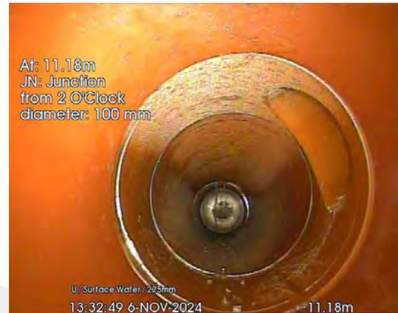
15.jpg, 00:00:58, 11.18 m Junction at 2 o'clock, diameter: 100mm
