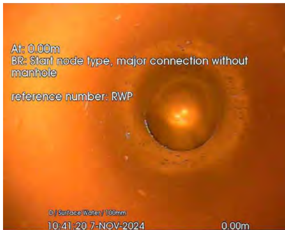
190.jpg, 00:00:01, 0.00 m Start node, major connection without manhole, reference: RWP
