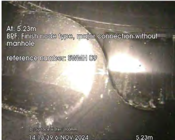
59.jpg, 00:00:28, 5.23 m Finish node, major connection without manhole, reference: SWMH 09
