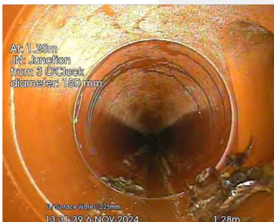
12.jpg, 00:00:17, 1.28 m Junction at 3 o'clock, diameter: 150mm
