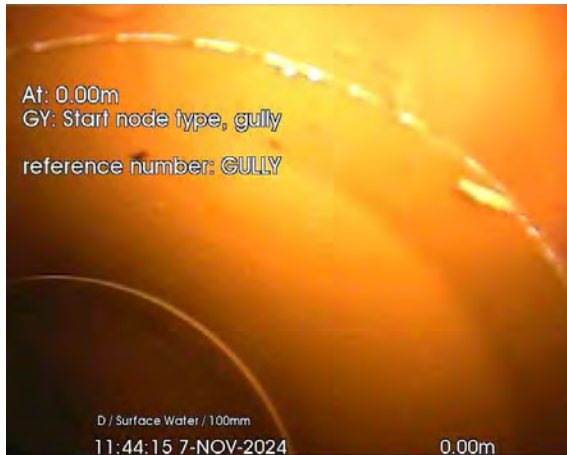
239.jpg, 00:00:00, 0.00 m Start node, gully, reference: GULLY
