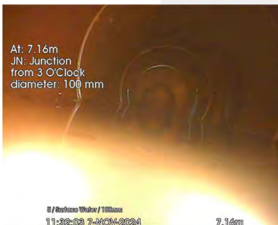
224.jpg, 00:00:37, 7.16 m Junction at 3 o'clock, diameter: 100mm
