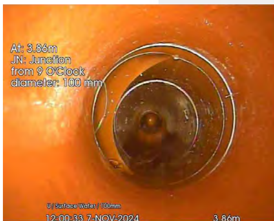
257.jpg, 00:00:16, 3.86 m Junction at 9 o'clock, diameter: 100mm
