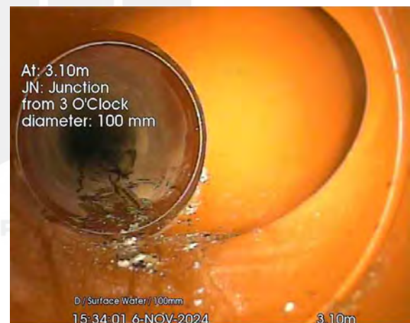
116.jpg, 00:00:14, 3.10 m Junction at 3 o'clock, diameter: 100mm
