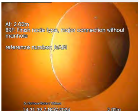
326.jpg, 00:00:23, 2.02 m Finish node, major connection without manhole, reference: MAIN
