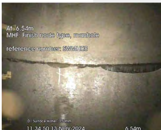
380.jpg, 00:00:20, 6.54 m Finish node, manhole, reference: SWMH08
