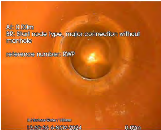
27.jpg, 00:00:01, 0.02 m Start node, major connection without manhole, reference: RWP
