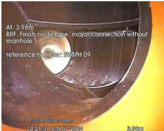
68.jpg, 00:00:28, 3.98 m Finish node, major connection without manhole, reference: SWMH 09
