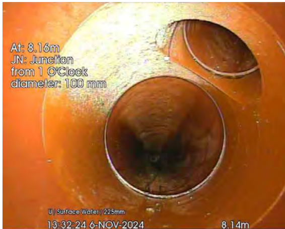
14.jpg, 00:00:45, 8.14 m Junction at 1 o'clock, diameter: 100mm
