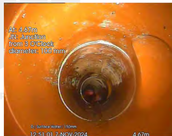
292.jpg, 00:00:28, 4.67 m Junction at 3 o'clock, diameter: 100mm
