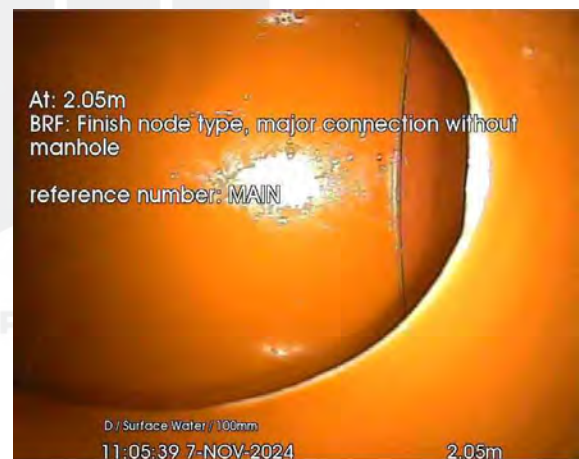
209.jpg, 00:00:19, 2.05 m Finish node, major connection without manhole, reference: MAIN
