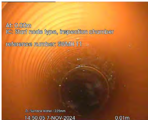
347.jpg, 00:00:01, 0.01 m Start node, inspection chamber, reference: SWMH 11
