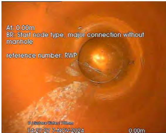
319.jpg, 00:00:00, 0.00 m Start node, major connection without manhole, reference: RWP
