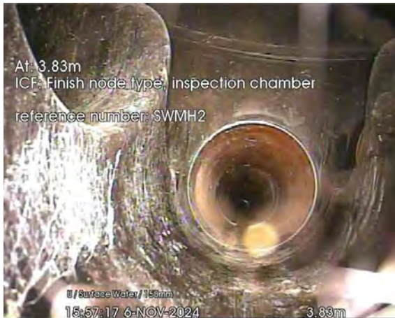
148.jpg, 00:00:23, 3.83 m Finish node, inspection chamber, reference: SWMH2
