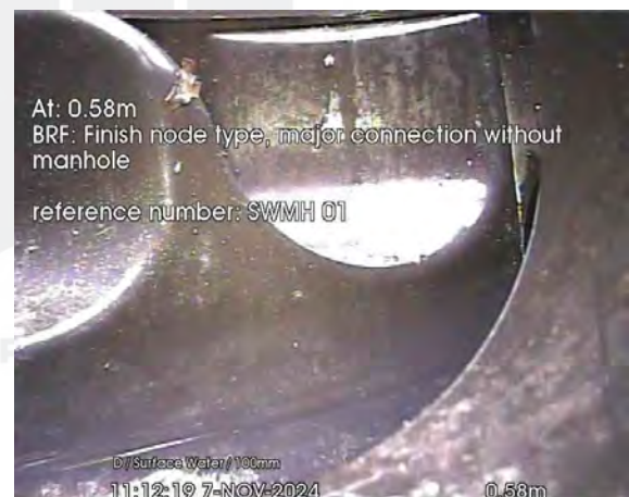
217.jpg, 00:00:13, 0.58 m Finish node, major connection without manhole, reference: SWMH 01
