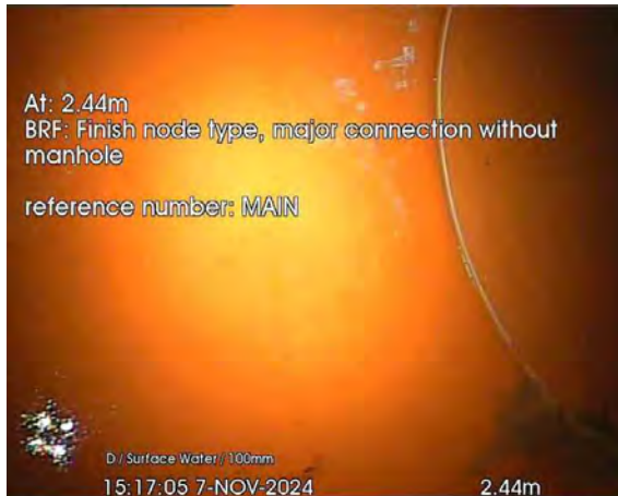
374.jpg, 00:00:23, 2.44 m Finish node, major connection without manhole, reference: MAIN
