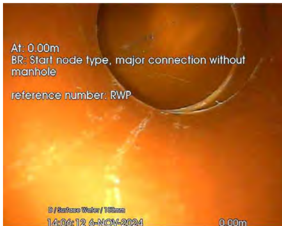
47.jpg, 00:00:02, 0.00 m Start node, major connection without manhole, reference: RWP
