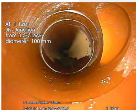
77.jpg, 00:00:11, 1.12 m Junction at 3 o'clock, diameter: 100mm
