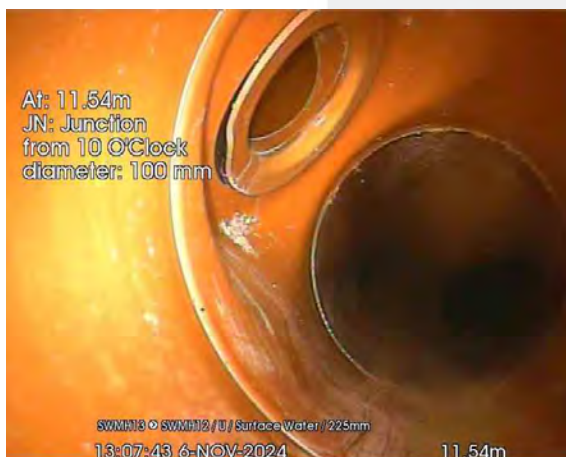
3.jpg, 00:00:40, 11.54 m Junction at 10 o'clock, diameter: 100mm
