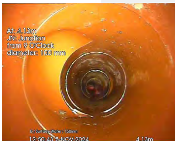
291.jpg, 00:00:21, 4.13 m Junction at 9 o'clock, diameter: 100mm
