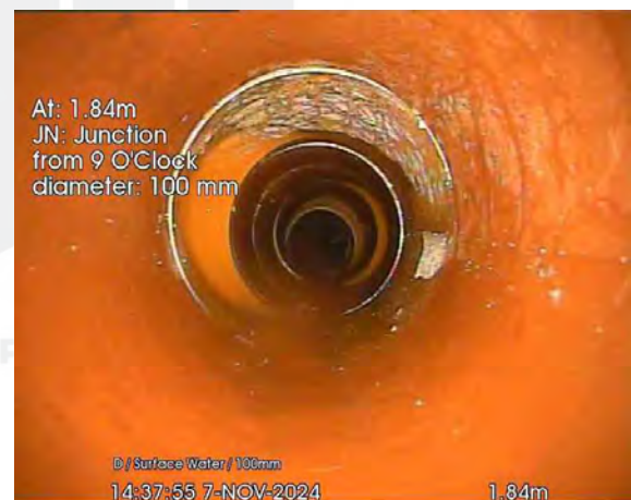
334.jpg, 00:00:11, 1.84 m Junction at 9 o'clock, diameter: 100mm
