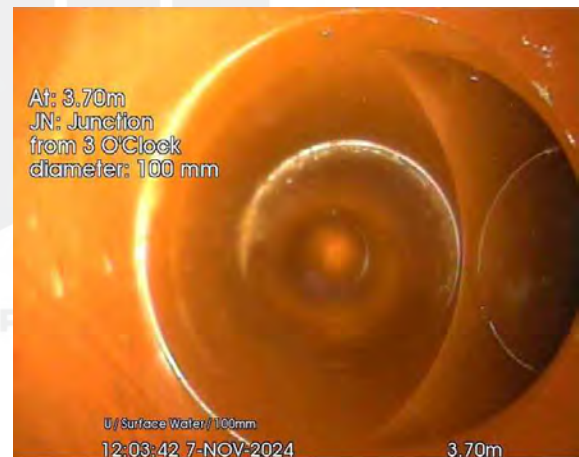
264.jpg, 00:00:20, 3.70 m Junction at 3 o'clock, diameter: 100mm
