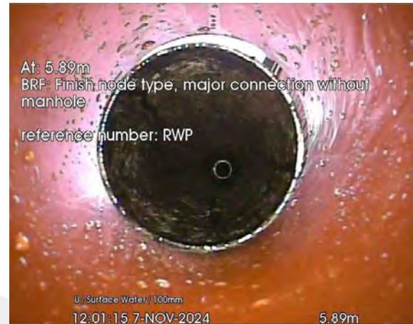
260.jpg, 00:00:33, 5.89 m Finish node, major connection without manhole, reference: RWP
