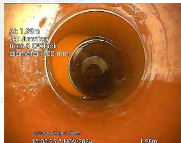
362.jpg, 00:00:11, 1.98 m Junction at 9 o'clock, diameter: 100mm
