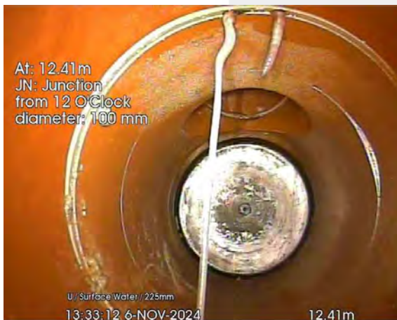
16.jpg, 00:01:09, 12.41 m Junction at 12 o'clock, diameter: 100mm
