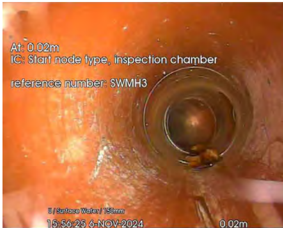
144.jpg, 00:00:00, 0.02 m Start node, inspection chamber, reference: SWMH3
