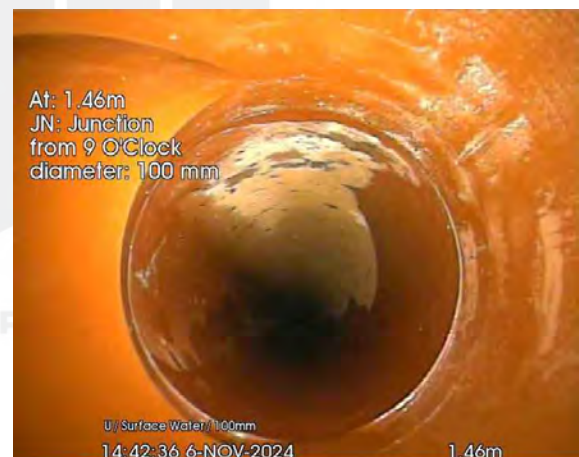
95.jpg, 00:00:18, 1.46 m Junction at 9 o'clock, diameter: 100mm
