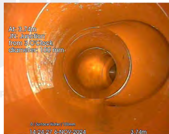
72.jpg, 00:00:26, 3.74 m Junction at 3 o'clock, diameter: 100mm
