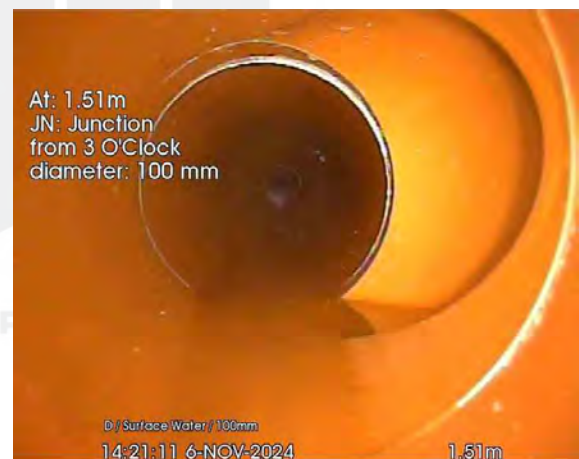
67.jpg, 00:00:15, 1.51 m Junction at 3 o'clock, diameter: 100mm
