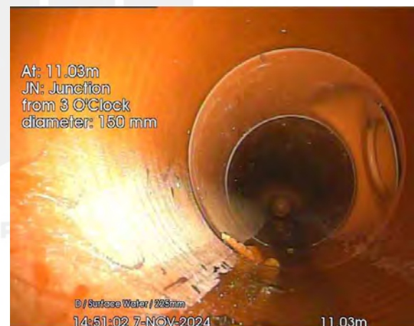
350.jpg, 00:00:29, 11.03 m Junction at 3 o'clock, diameter: 150mm
