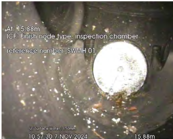
202.jpg, 00:00:46, 15.88 m Finish node, inspection chamber, reference: SWMH 01
