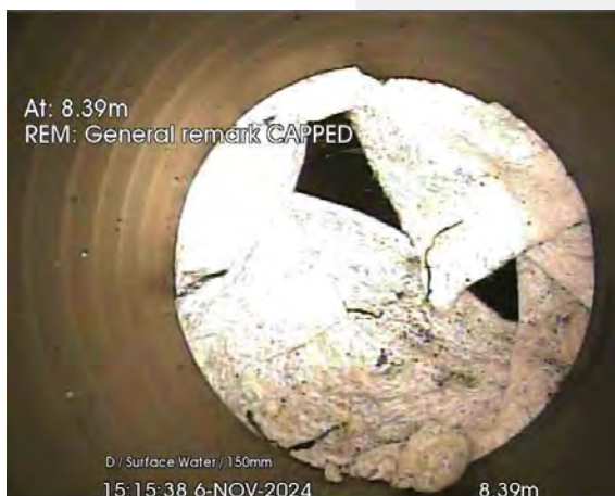
108.jpg, 00:00:30, 8.39 m General remark, CAPPED
