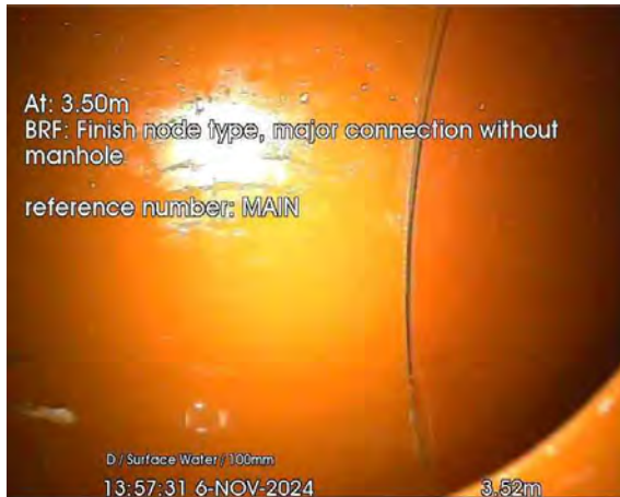
42.jpg, 00:00:25, 3.52 m Finish node, major connection without manhole, reference: MAIN
