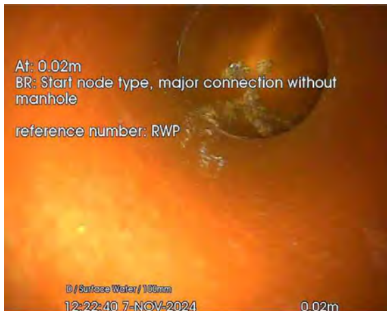
279.jpg, 00:00:02, 0.02 m Start node, major connection without manhole, reference: RWP
