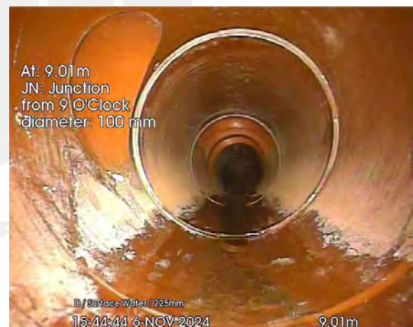
129.jpg, 00:00:32, 9.01 m Junction at 9 o'clock, diameter: 100mm
