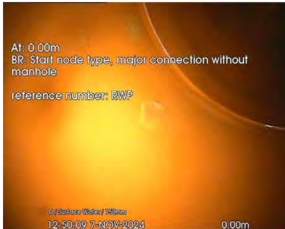
289.jpg, 00:00:04, 0.00 m Start node, major connection without manhole, reference: RWP
