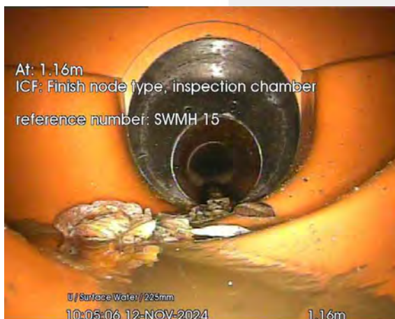
377.jpg, 00:00:20, 1.16 m Finish node, inspection chamber, reference: SWMH 15
