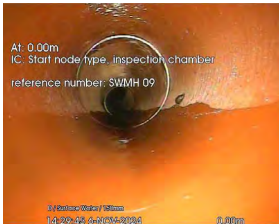
75.jpg, 00:00:02, 0.00 m Start node, inspection chamber, reference: SWMH 09
