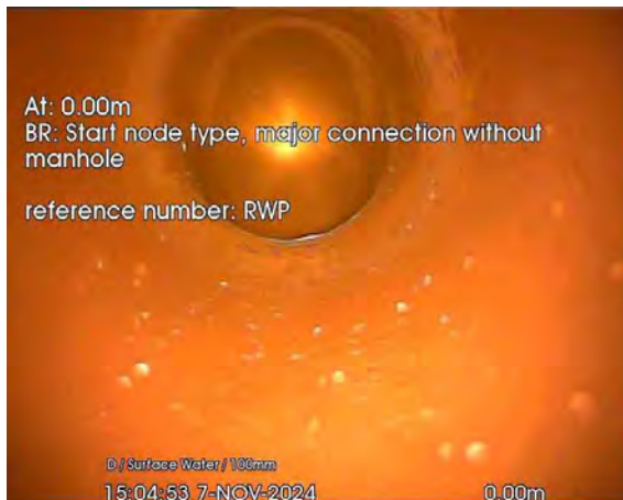
359.jpg, 00:00:00, 0.00 m Start node, major connection without manhole, reference: RWP
