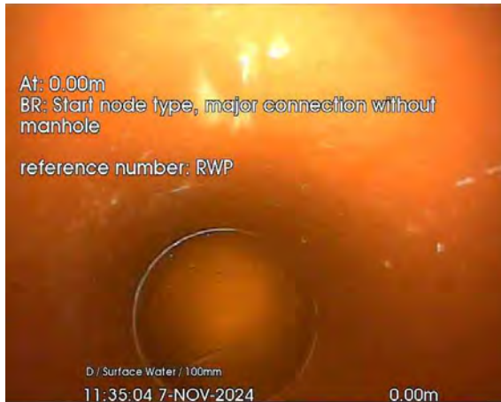
227.jpg, 00:00:03, 0.00 m Start node, major connection without manhole, reference: RWP
