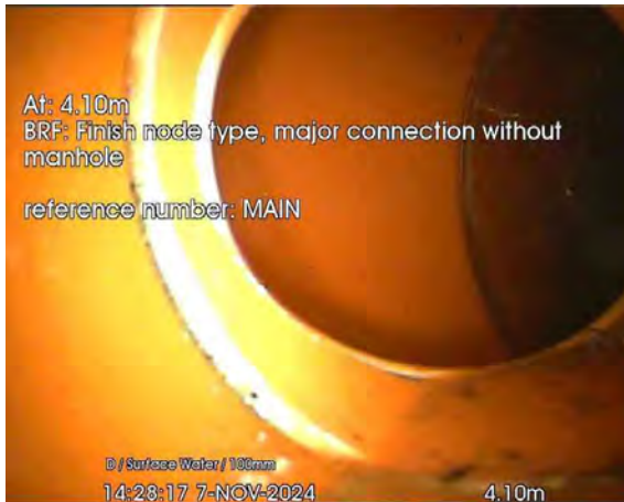
323.jpg, 00:00:23, 4.10 m Finish node, major connection without manhole, reference: MAIN
