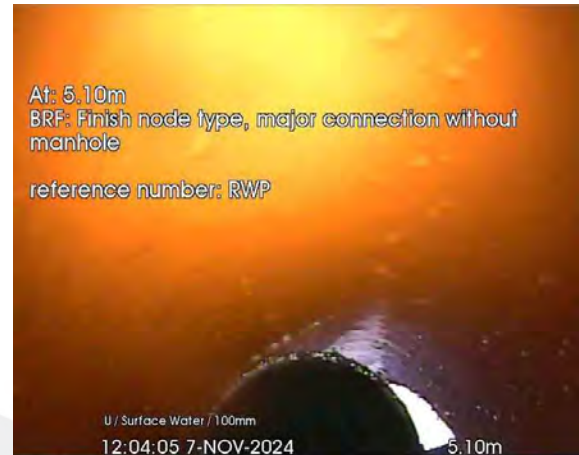
266.jpg, 00:00:31, 5.10 m Finish node, major connection without manhole, reference: RWP
