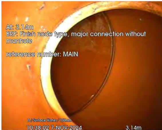
189.jpg, 00:00:32, 3.14 m Finish node, major connection without manhole, reference: MAIN
