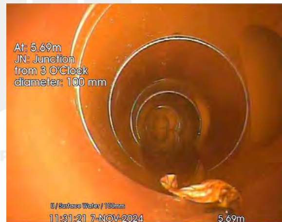
221.jpg, 00:00:20, 5.69 m Junction at 3 o'clock, diameter: 100mm
