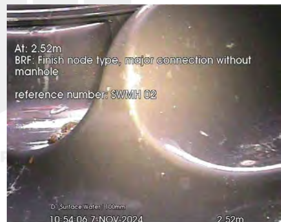
197.jpg, 00:00:17, 2.52 m Finish node, major connection without manhole, reference: SWMH 02
