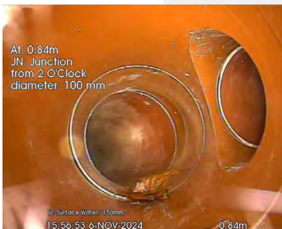
146.jpg, 00:00:10, 0.84 m Junction at 2 o'clock, diameter: 100mm
