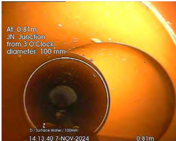
309.jpg, 00:00:17, 0.81 m Junction at 3 o'clock, diameter: 100mm
