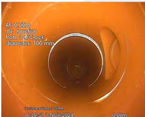
220.jpg, 00:00:04, 0.00 m Junction at 3 o'clock, diameter: 100mm
