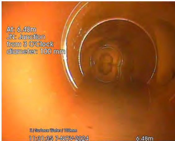
222.jpg, 00:00:25, 6.48 m Junction at 3 o'clock, diameter: 100mm
