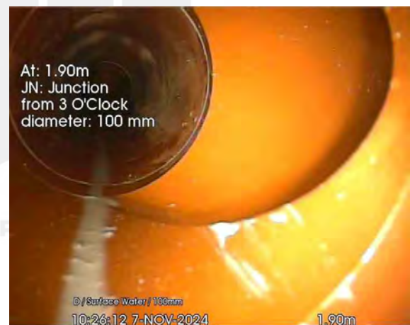
174.jpg, 00:00:20, 1.90 m Junction at 3 o'clock, diameter: 100mm
