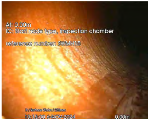
7.jpg, 00:00:01, 0.00 m Start node, inspection chamber, reference: SWMH15
