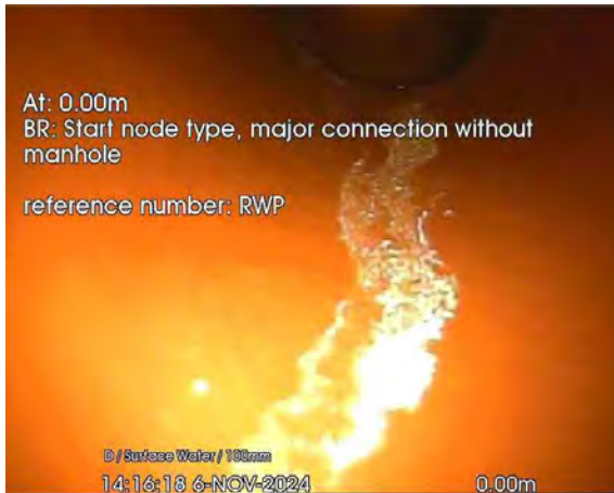
60.jpg, 00:00:01, 0.00 m Start node, major connection without manhole, reference: RWP
