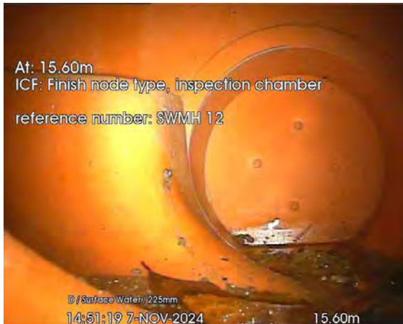
351.jpg, 00:00:39, 15.60 m Finish node, inspection chamber, reference: SWMH 12
