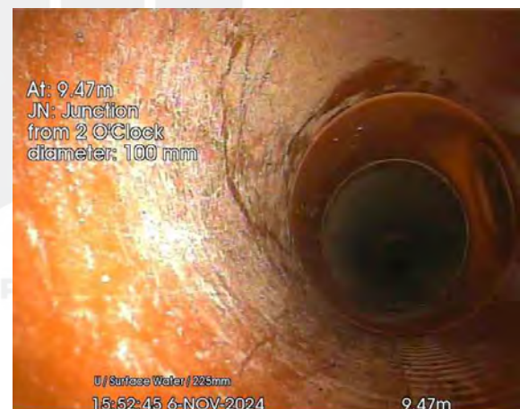
142.jpg, 00:00:22, 9.47 m Junction at 2 o'clock, diameter: 100mm
