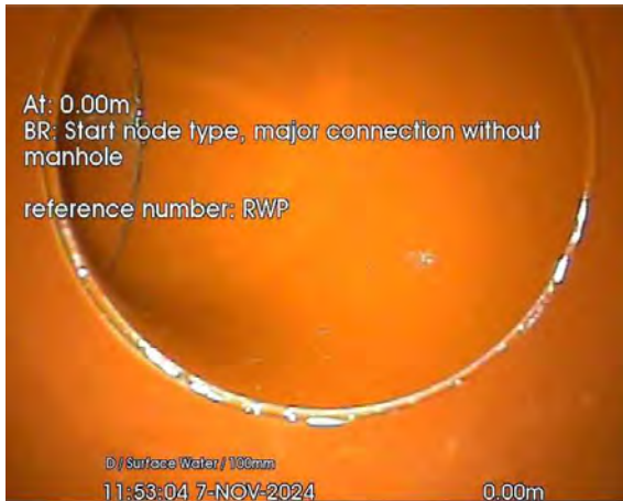
247.jpg, 00:00:01, 0.00 m Start node, major connection without manhole, reference: RWP
