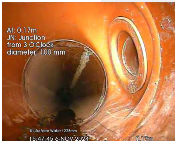
133.jpg, 00:00:04, 0.17 m Junction at 3 o'clock, diameter: 100mm
