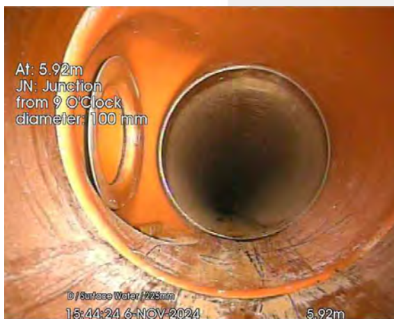
128.jpg, 00:00:23, 5.92 m Junction at 9 o'clock, diameter: 100mm
