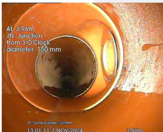
299.jpg, 00:00:12, 3.96 m Junction at 3 o'clock, diameter: 150mm
