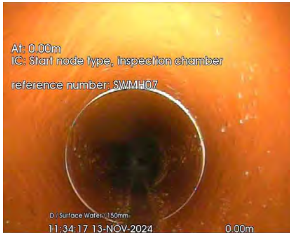
378.jpg, 00:00:00, 0.00 m Start node, inspection chamber, reference: SWMH07
