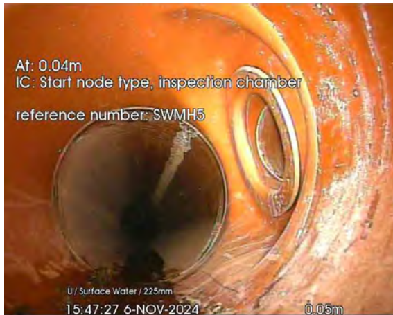
131.jpg, 00:00:00, 0.05 m Start node, inspection chamber, reference: SWMH5
