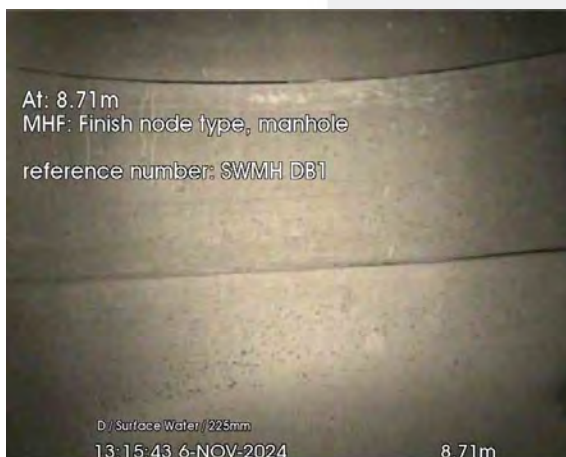
9.jpg, 00:00:29, 8.71 m Finish node, manhole, reference: SWMH DB1
