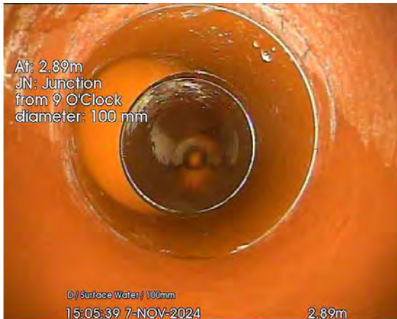
363.jpg, 00:00:16, 2.89 m Junction at 9 o'clock, diameter: 100mm
