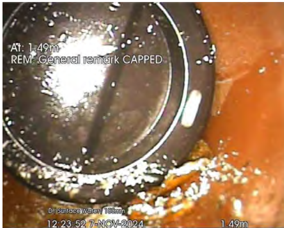
283.jpg, 00:00:20, 1.49 m General remark, CAPPED
