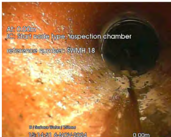
106.jpg, 00:00:02, 0.00 m Start node, inspection chamber, reference: SWMH 18
