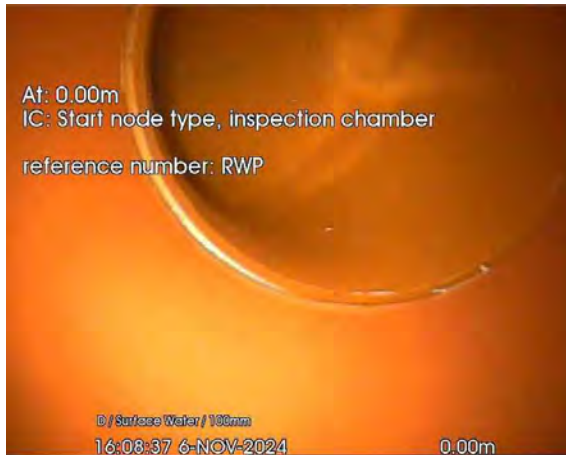
149.jpg, 00:00:00, 0.00 m Start node, inspection chamber, reference: RWP
