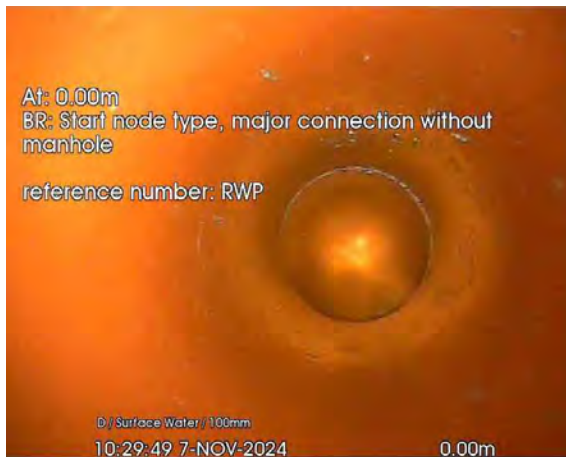
176.jpg, 00:00:04, 0.00 m Start node, major connection without manhole, reference: RWP
