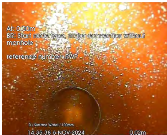
84.jpg, 00:00:01, 0.02 m Start node, major connection without manhole, reference: RWP
