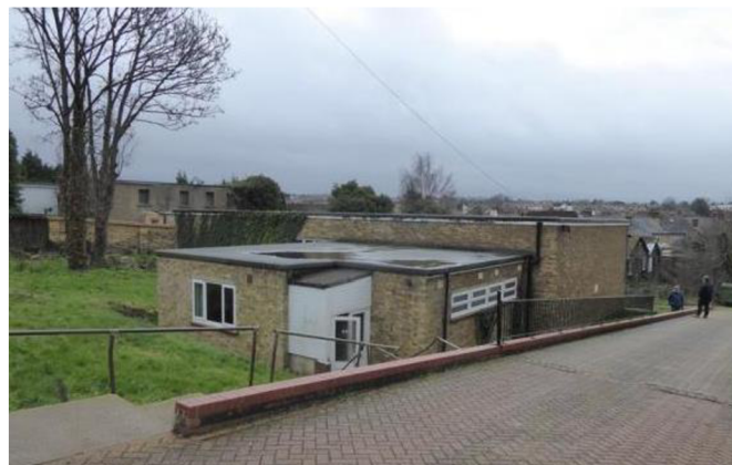
Above Right: Vehicle Access ramp to Wycliffe House
