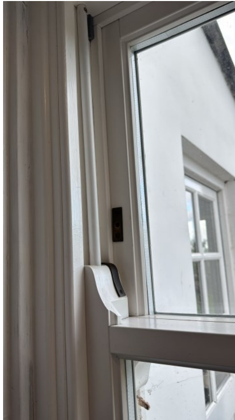
Fig .6. Close up photo of kitchen window
