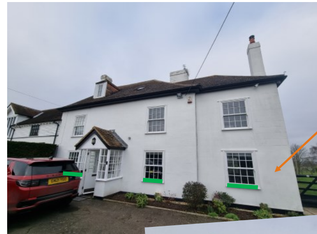
Fig .2. Original window openings
