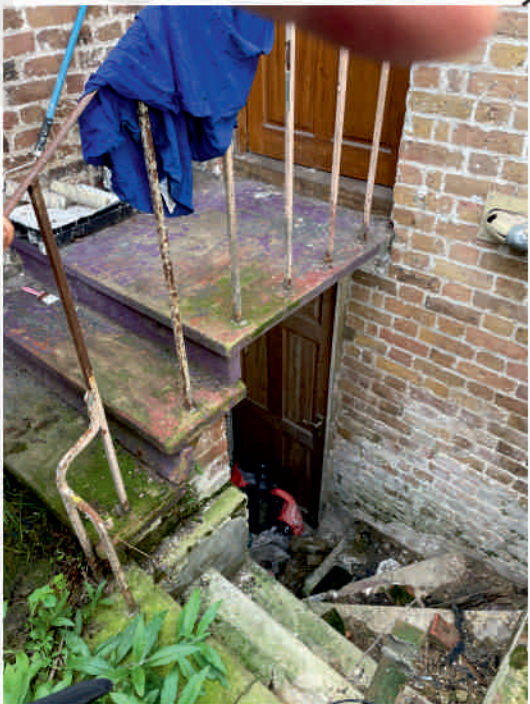
PHOTOGRAPH 1 Showing original rear steps from first floor to ground floor to probably former coal hole
