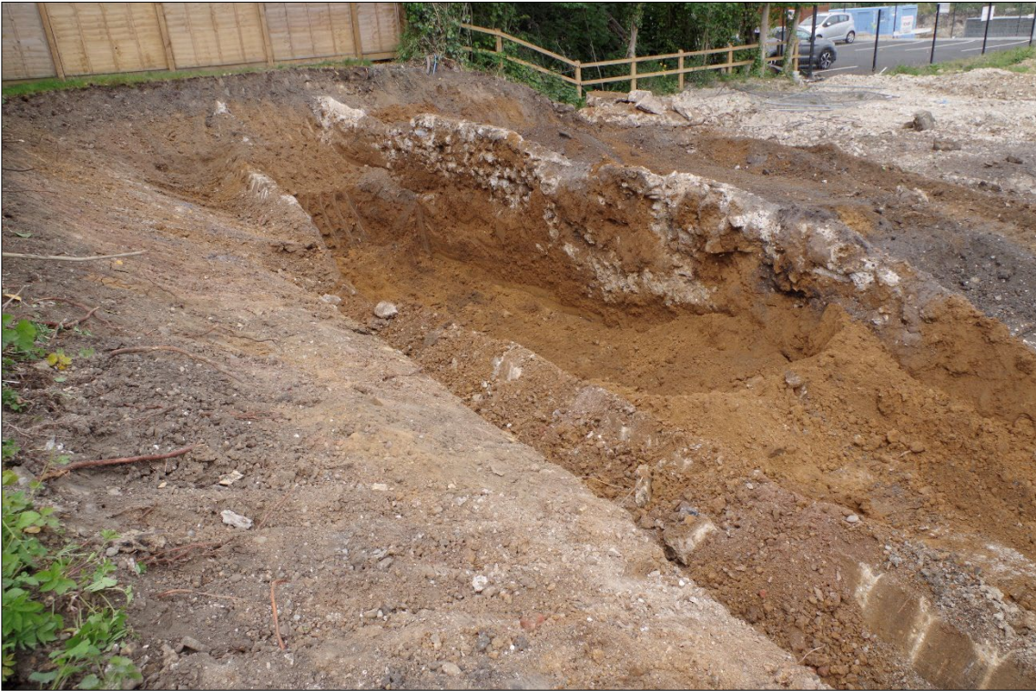
Exposed walls from the southeast
