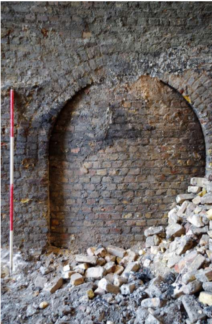
Plate 5 Intricately bricked up openings at the floor of the kiln tunnel
