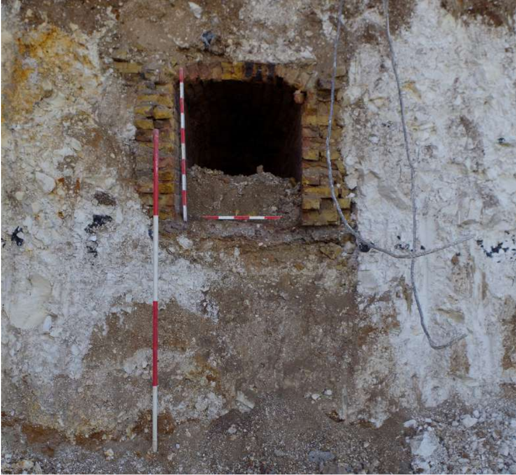
Plate 21 The Adit or 'pedestrian' tunnel in the chalk face, viewed from the northeast
