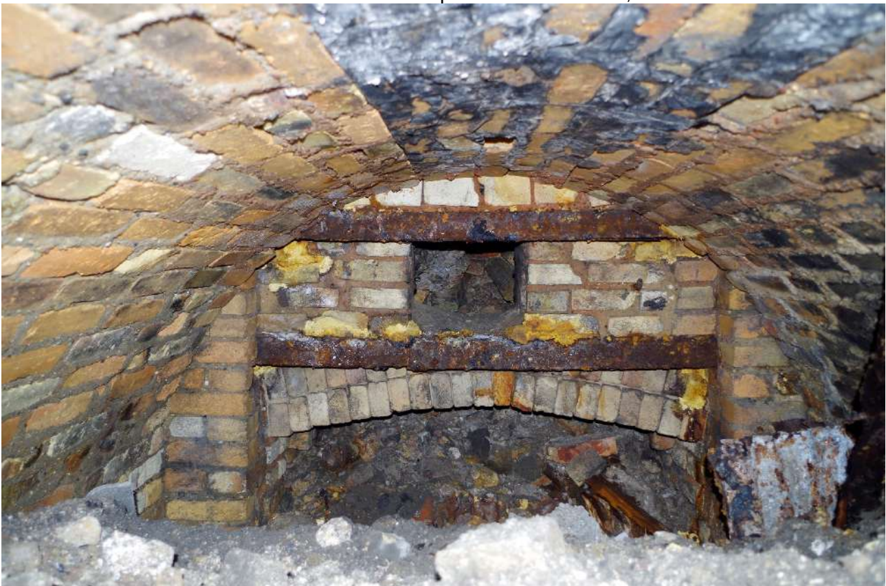
Plate 18 The fire box and a stoke hole at the base of the kiln
