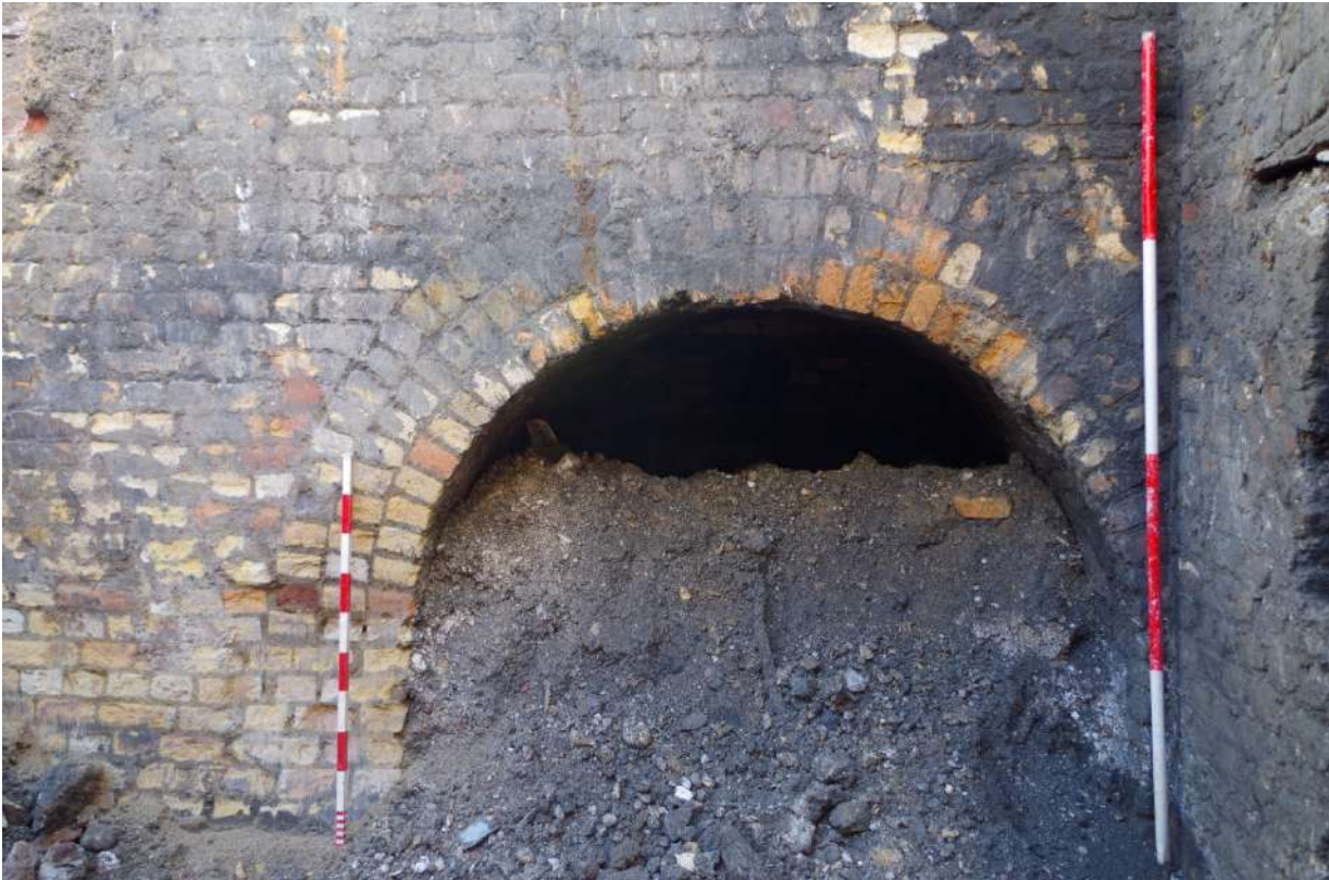
Plate 17 The draw door at the base of the open section of tunnel, viewed from the east
