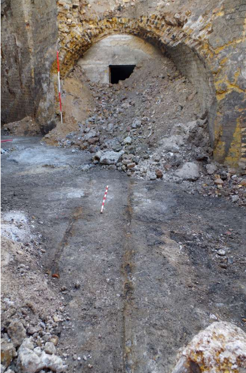
Plate 19 The southwestern section of Tunnel 22A, its associated (later) railway tracks are visible at the base of the open section of tunnel, viewed from the northeast
