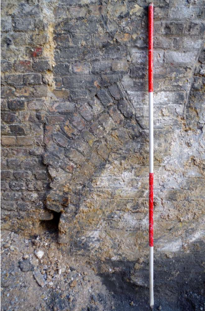
Plate 20 Bricked up draw door to allow for the insertion of tunnel 22A, viewed from the east
