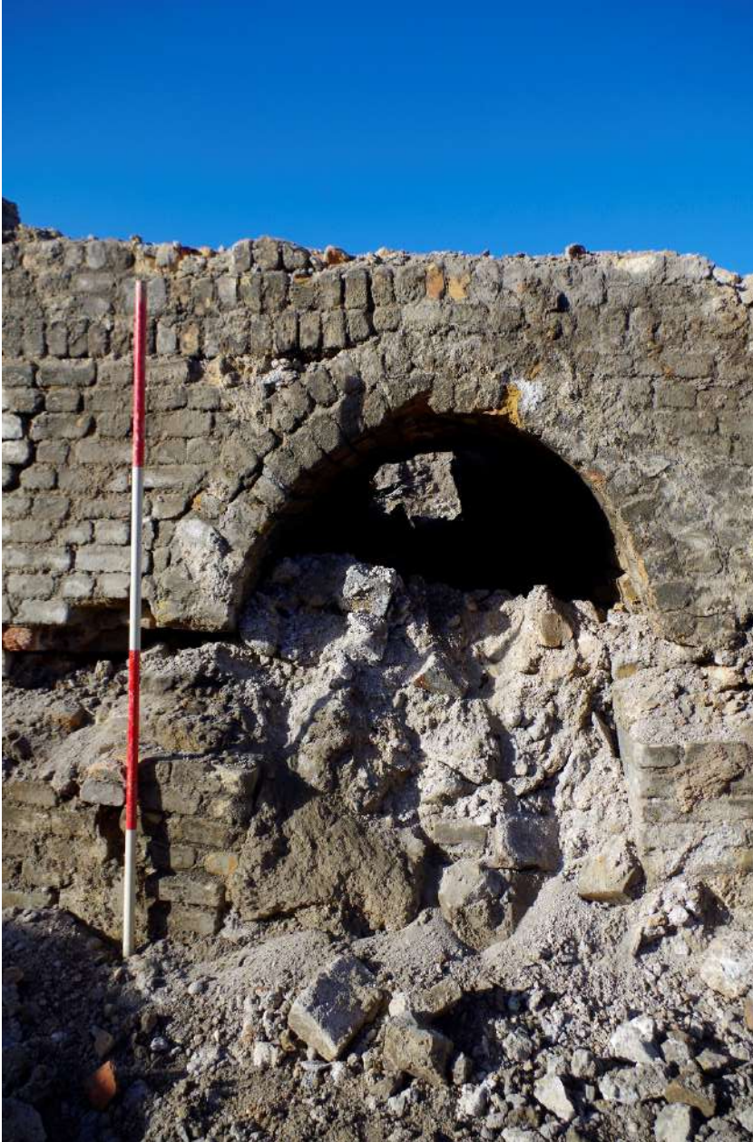
Plate 16 Loading chamber for the remaining kiln on the western side of the tunnel
