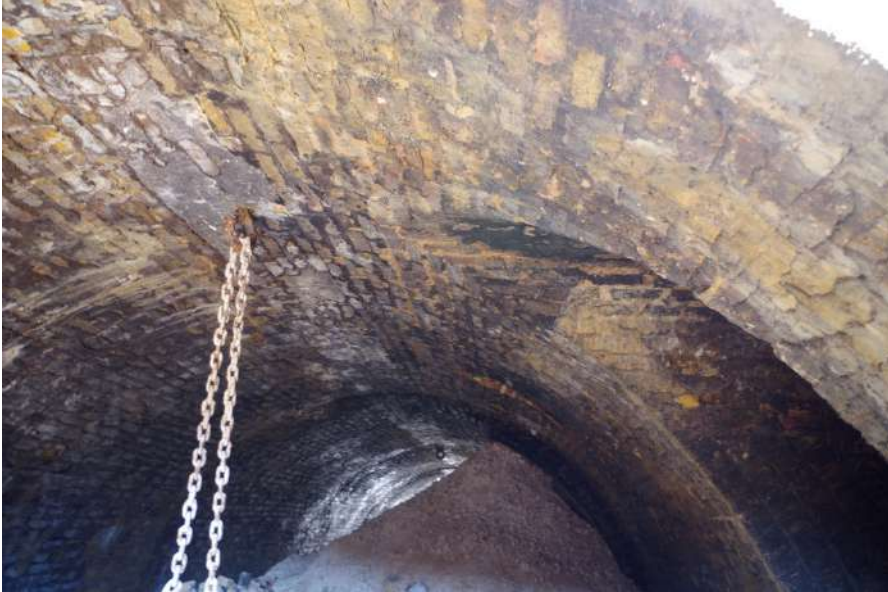
Plate 4 Metal hoop set at the crown of the tunnel for use in loading chambers
