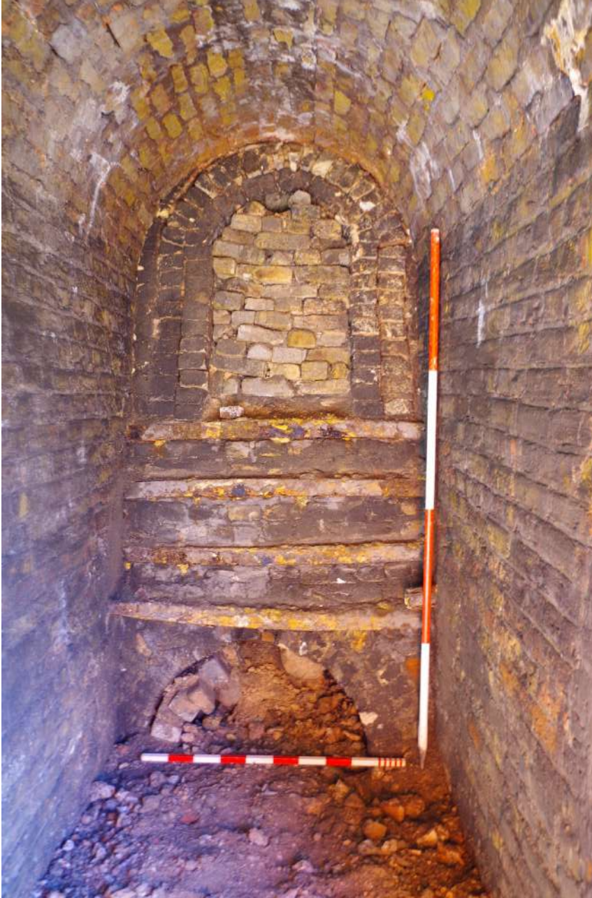
Plate 7 The Kiln loading doors
