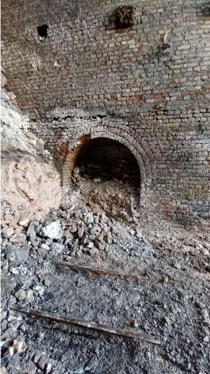
Plate 3 Interior of the kiln tunnel, with railway tracks at base, niche/recess in the side wall and first floor flooring joists.
