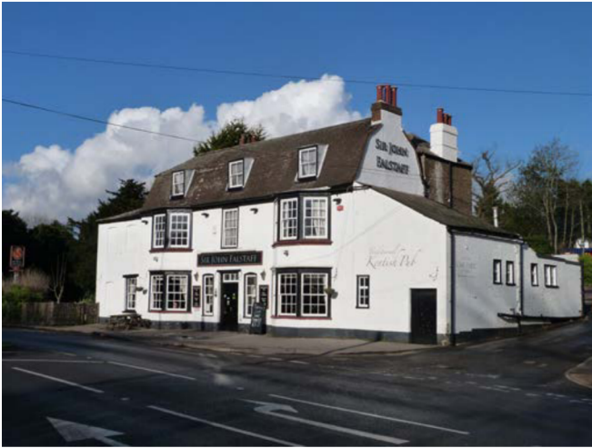
Plate 1 South western elevation showing original phase constructed in painted brick. The gambrel style roof is visible in this view.
