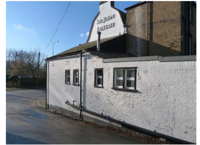
Plate 6 Single storey lean to and flat roof type additions to the south.
