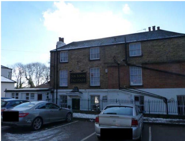
Plate 5 North eastern elevation showing an area which has been rebuilt in red brick.
