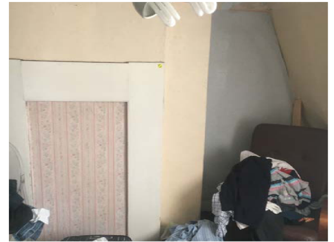
Plate 12 Attic level room.
