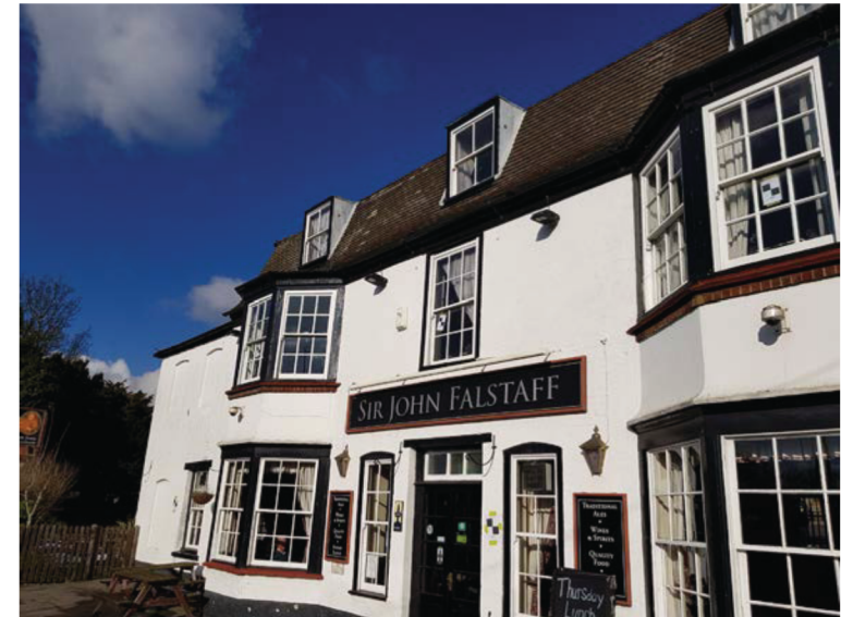
Plate 13 South western, principal elevation.
