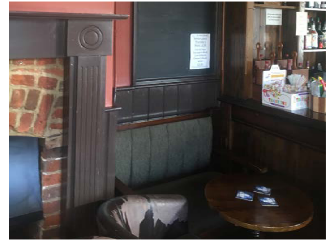
Plate 9 View of retained chimney breast with modern insert and mantle.
