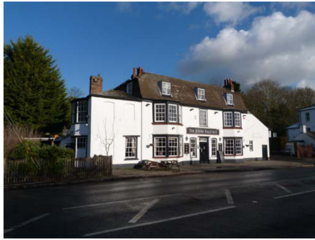
Plate 2 South western elevation showing side addition.
