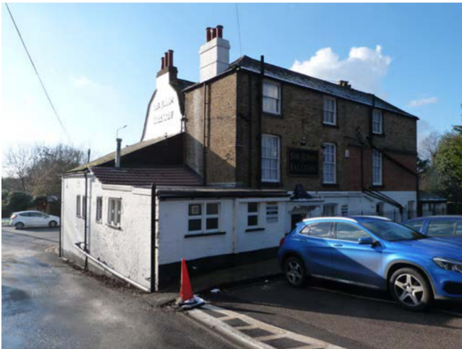
Plate 4 View showing 19th century full height rear extension constructed in yellow stock brick.
