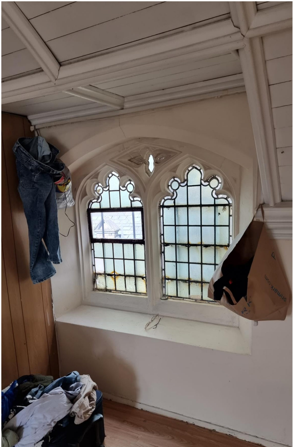
Fig.12: The former balcony to the chapel, now the mezzanine bedroom (room 25) with tracery window, barrel vaulted ceiling, and modern partition wall (left) to form the room.
