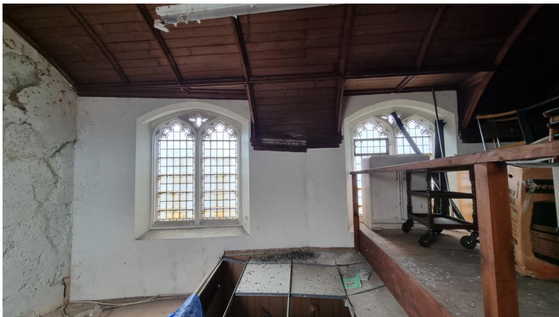
Fig.11: The chapel to the rear of the building (room 18), constructed at some point between 1907-32.
