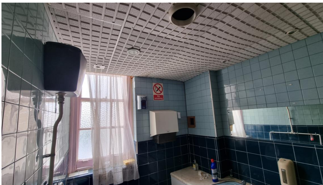
Fig.10: Modern first floor toilets (room 6).
