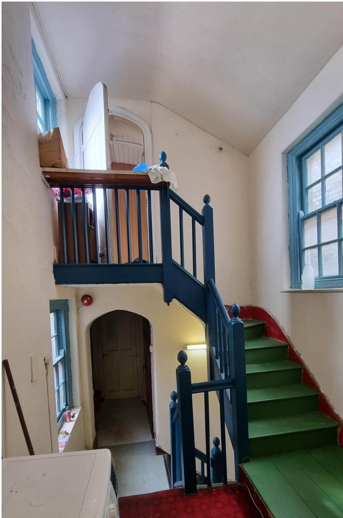
Fig.13: The early/mid-20 th century stairs between the chapel levels (room 20 of HS3 ). The windows to the left are into the lightwell (5) and the upper doorway leads to the mezzanine bedroom (room 25).
