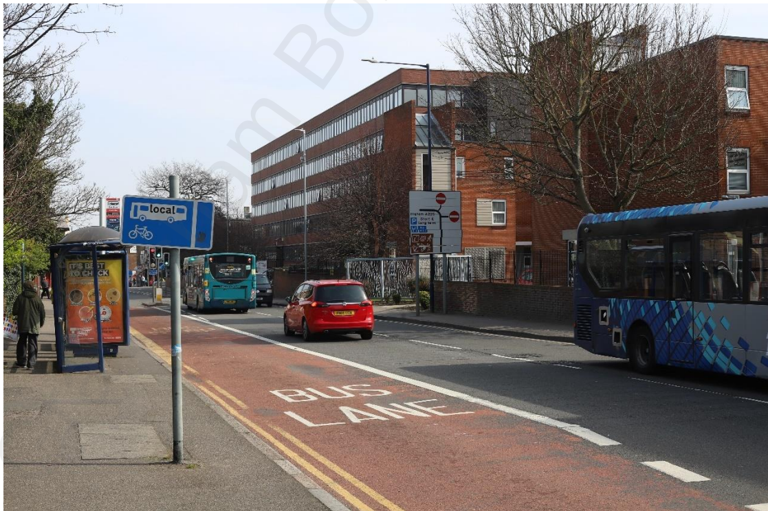
Plate 2 Joynes House, western and northern elevations.
