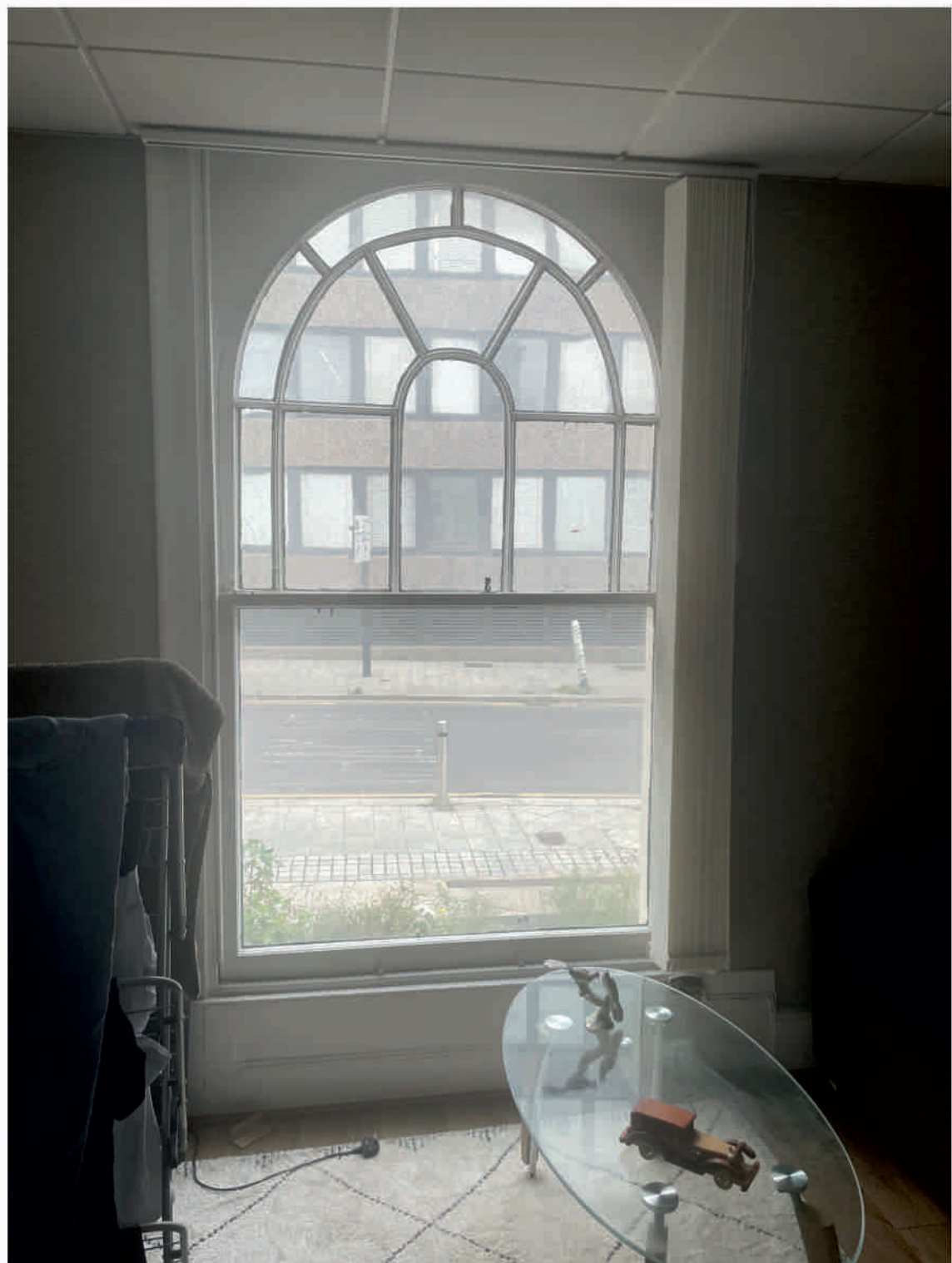
ROOM 1 - Original curved top sash window in good order to be made good. Note there are no window bars in the lower sash. Note suspended ceiling to room 1. Intention is to re bar the lower pane to match existing above and install secondary glazing (including room 2).
