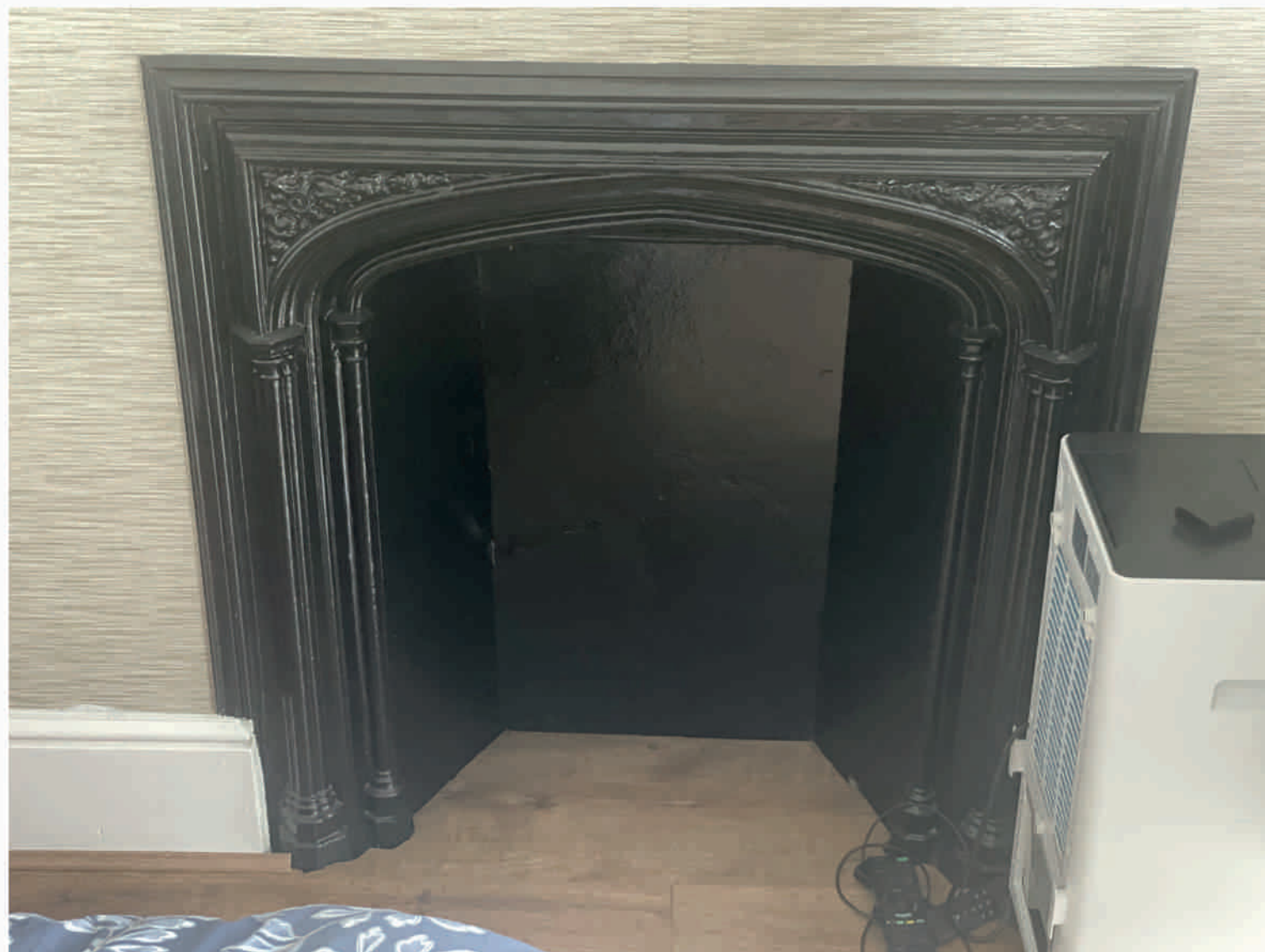
ROOM 1 - Central original fire place and surround to remain intact with replace skirting.
