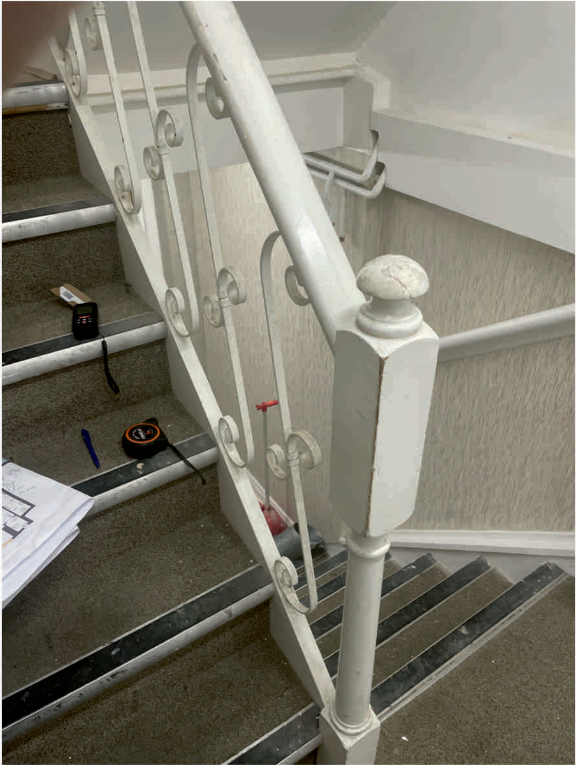
STAIR ENCLOSURE 5 - Showing original newel post and string to remain. No other original features remain.
