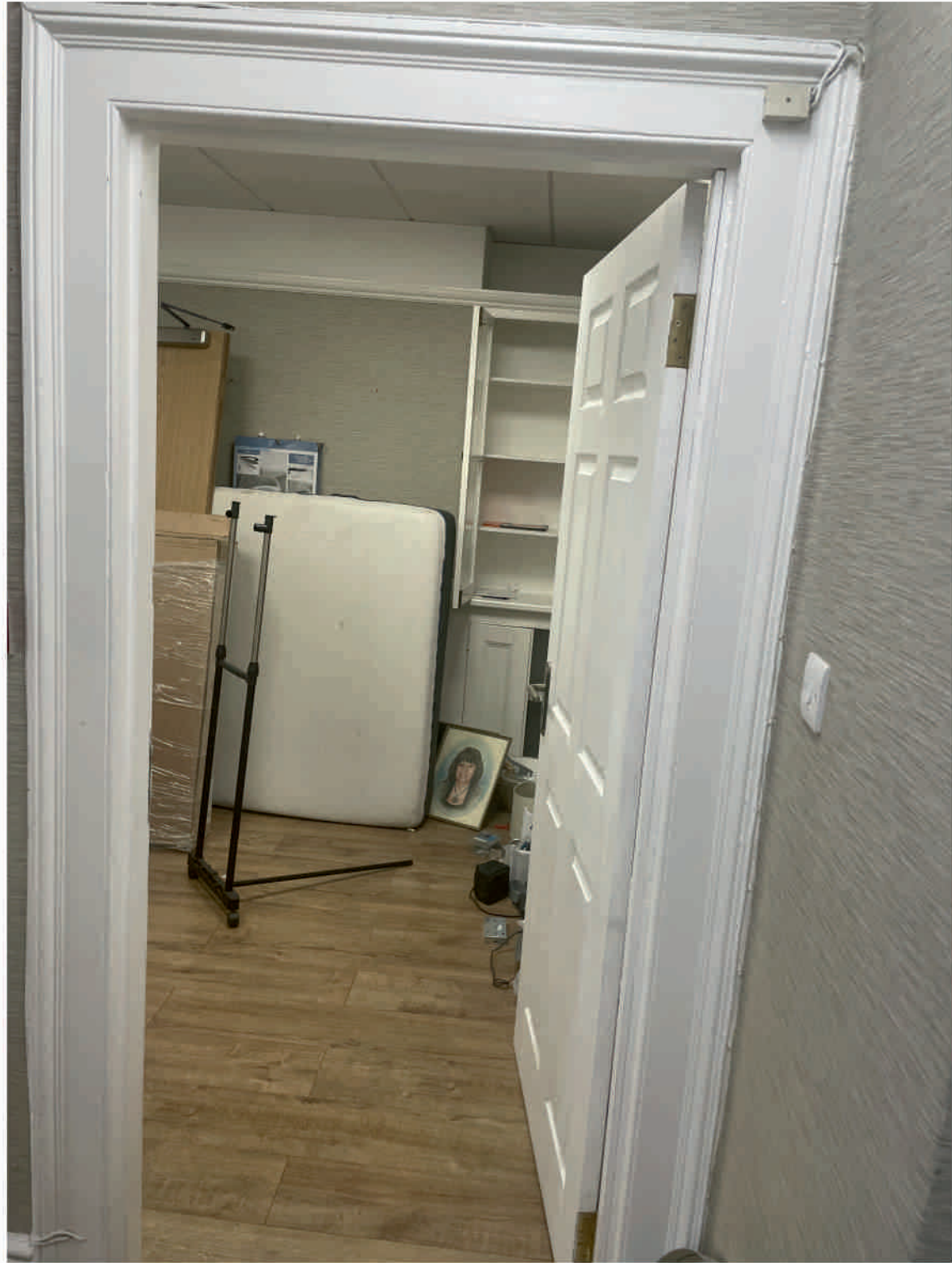
STAIR ENCLOSURE 5 - View into room 6 showing original frame and architrave with replacement 30min FR pressed door.
