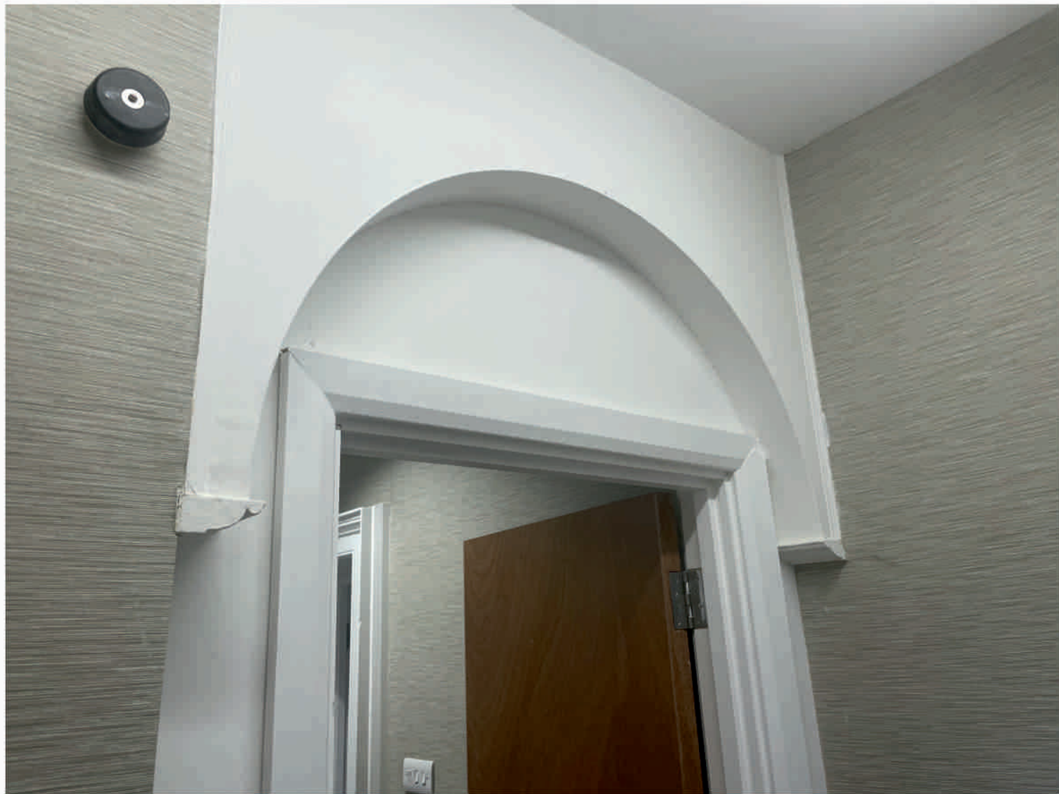
STAIR ENCLOSURE 5 - Looking toward lobby area 3. Original arch remains but with new partition and 30min FR door installed. No other original features.
