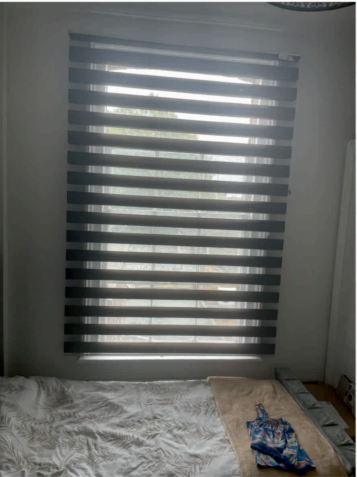
ROOM 19 - Showing original window behind blind (Broken would not move) with sash window bars in good order to be made good with internal secondary glazing. Original cornice remains intact.
