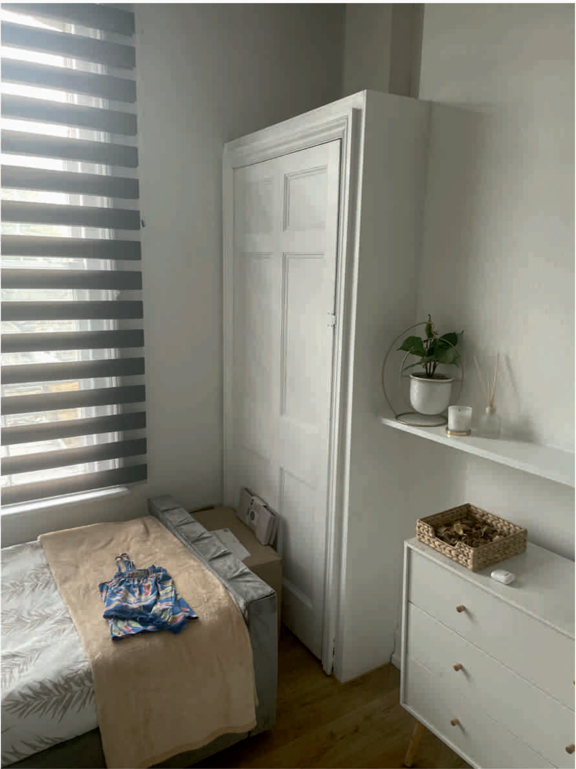
ROOM 19 - Original built in wardrobe and skirtings not no fireplace, surround .
