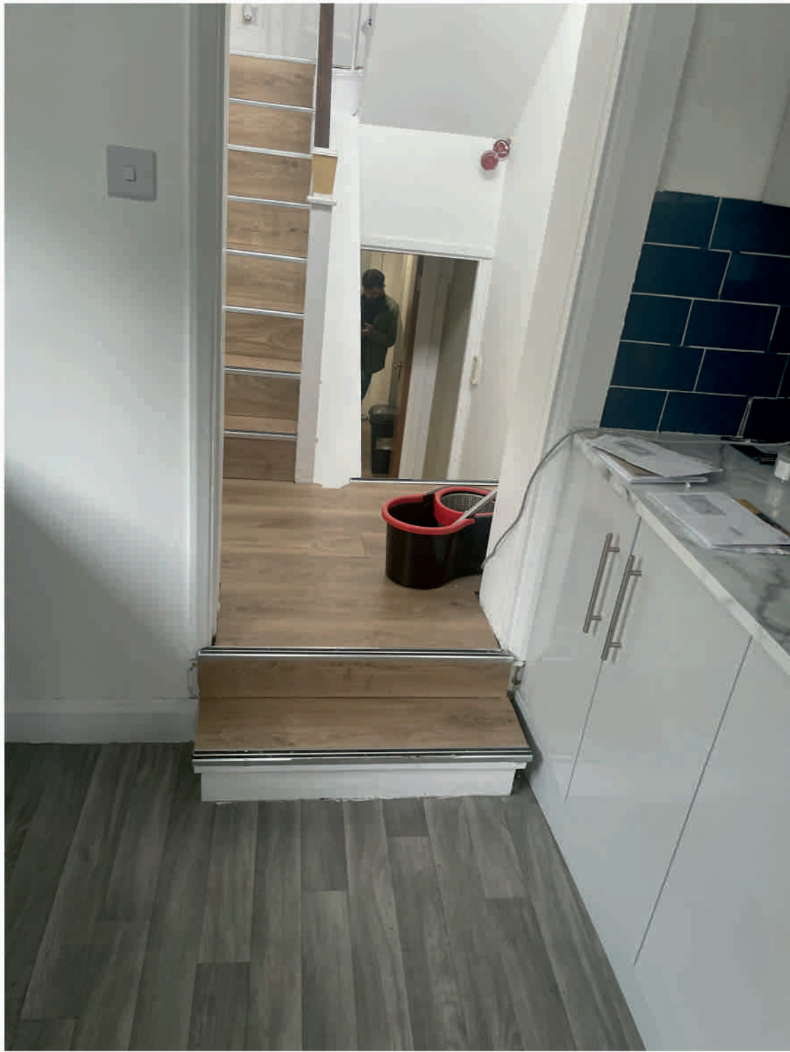
ROOM 16 - Looking back from room 169 toward entrance on to stair enclosure, No original features.
