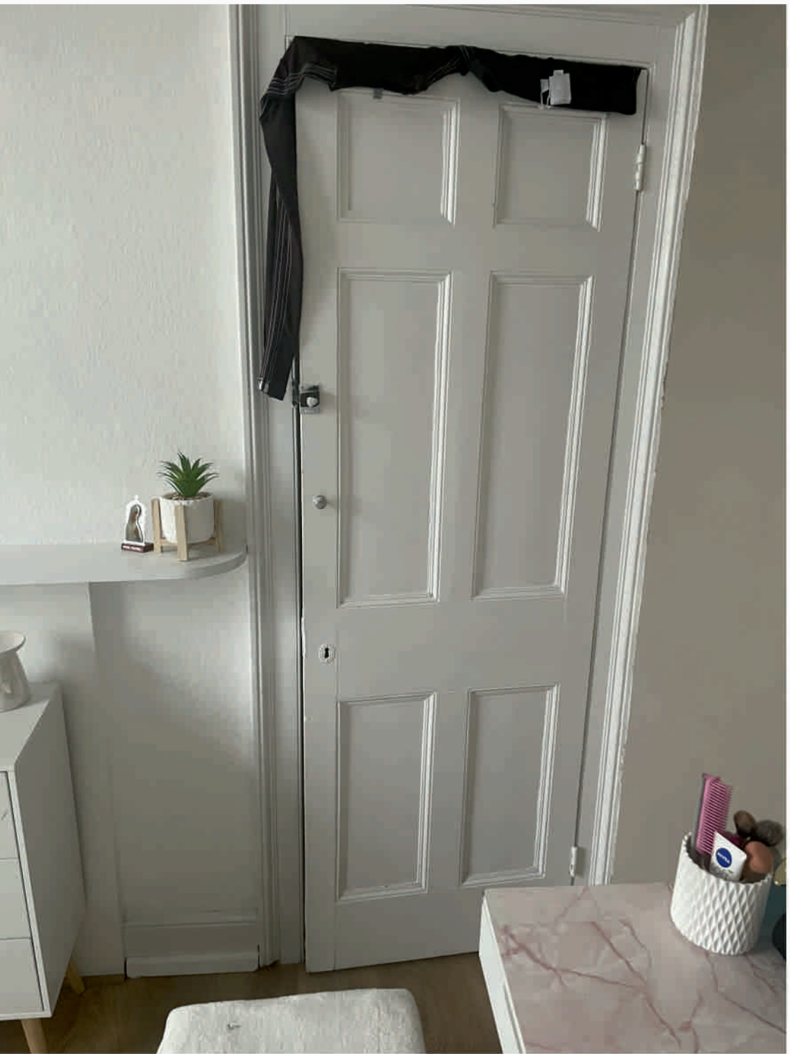
ROOM 19 - Original built in wardrobe and skirtings
